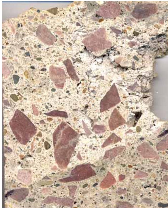
Figure 1. Example of a water–cement ratio anomaly in concrete from I-29 in western Iowa
