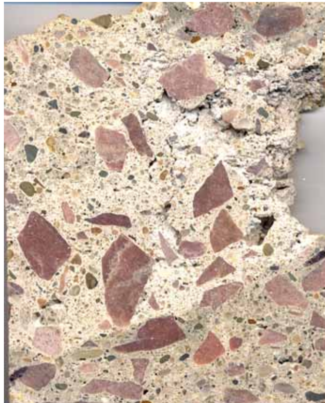
Figure 1. Example of a water–cement ratio anomaly in concrete from I-29 in western Iowa
