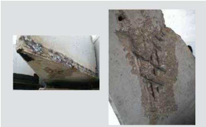
**Figure 1.** End damage observed on skewed bridge box beams during production.
