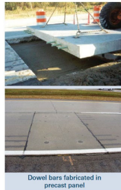
Dowel bars fabricated in precast panel
