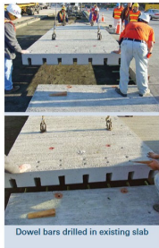
Dowel bars drilled in existing slab
