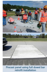
Precast panel using full dowel bar retrofit installation
