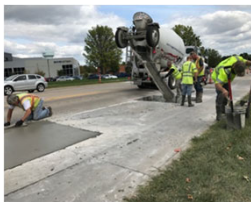
Full-Depth Repairs
