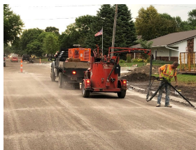
Joint/Crack Sealing
