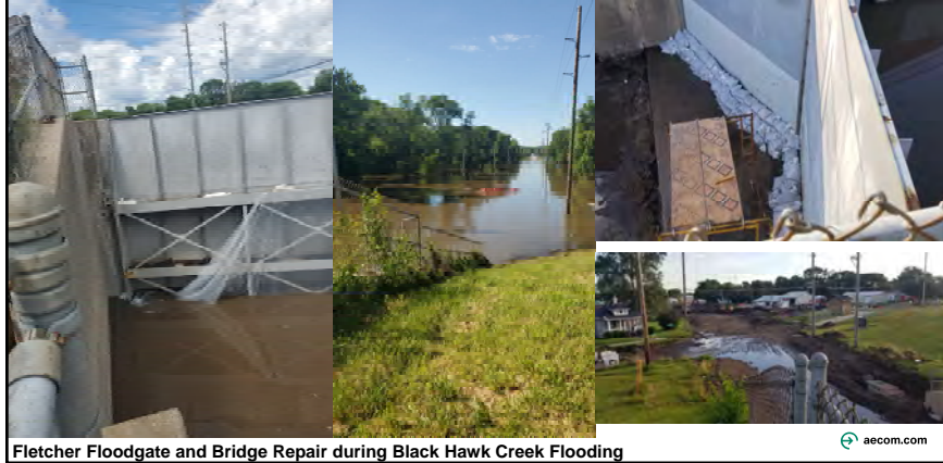
Fletcher Floodgate and Bridge Repair during Black Hawk Creek Flooding
