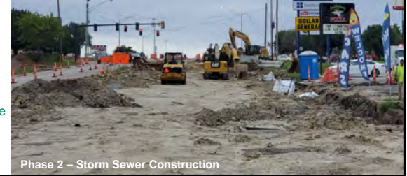
Phase 2 – Storm Sewer Construction
