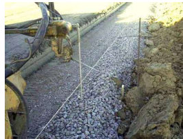
Stringline and paving hub alignment (from Minnesota DOT)
