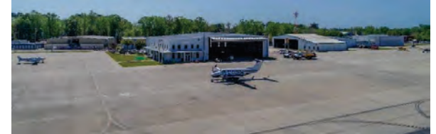
Grand Strand Ramp – Although not an overlay, the consultant did allow the aggregate base to be recycled back under the P-501
