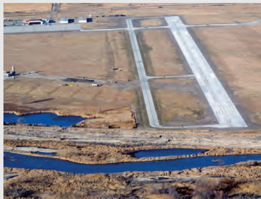
Concrete Overlay was less than 1/2 the cost of reconstruction!
