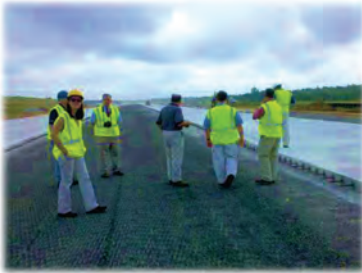
Lancaster County Airport Concrete Overlay of Asphalt
