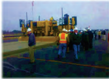
Charleston Exec Airport Concrete Overlay of Concrete
