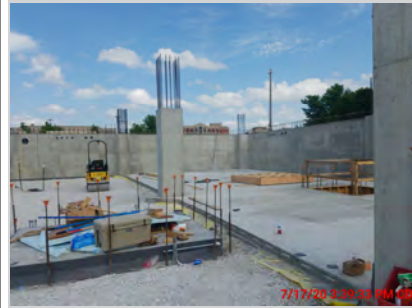
Left: Foundation walls and SOG Right: Birds Run Sewer Beams
