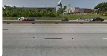
IH 10 in Houston, TX (2013) Photo: Andy Naranjo, TxDOT
