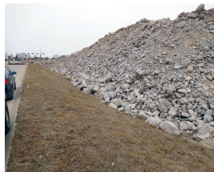
Photo: Dwayne Stenlund, MnDOT
