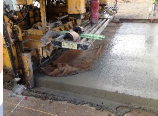
Placement of Concrete with Nano Silica
