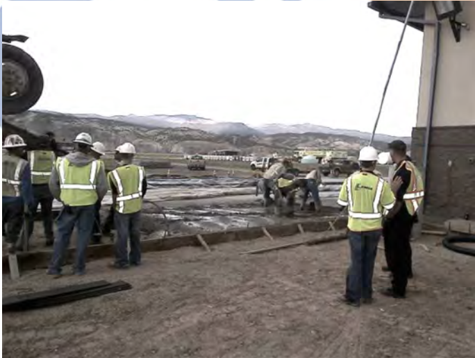
Placement of Nano Silica Concrete
