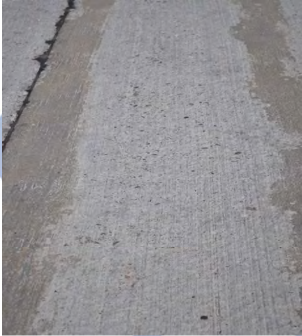
Standard Concrete Mix with Moderate to Extreme Surface Abrasive Wear
