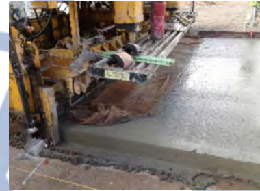
Placement of Nano Engineered Concrete
