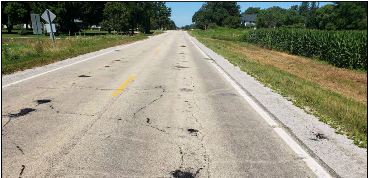
Existing Conditions: 12 in. AC Layer
