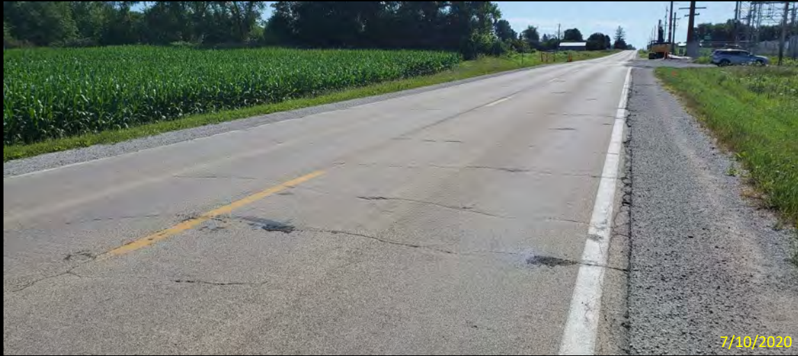
Existing Conditions: 12 in. AC Layer
