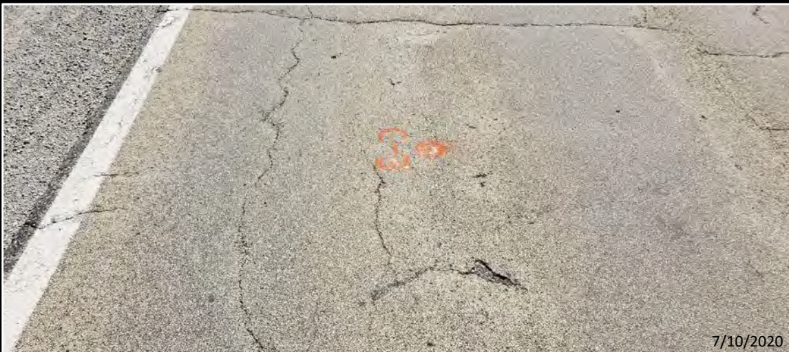
Existing Conditions: 12 in. AC Layer
