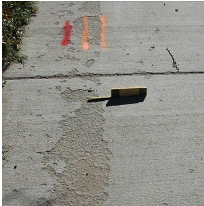
Figure 2. This pattern of scaling is more likely to be from differences in finishing.
