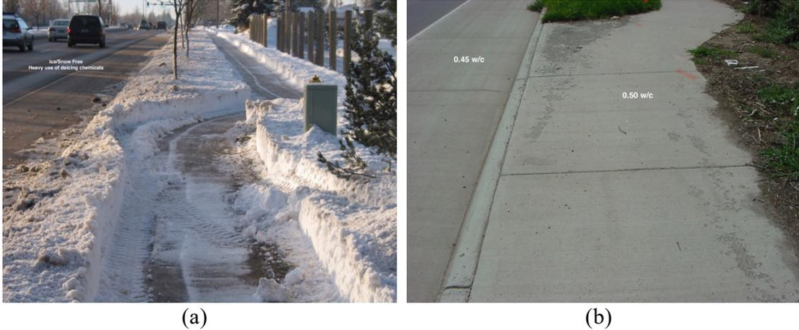
Figure 1. Winter (a), road heavily deiced and plowed. The snow/deicer from the road gets put on the sidewalk, which is kept open with a skid steer. Spring (b), scaling where snow was piled. The only difference between the concretes was the  $w/c$ .
