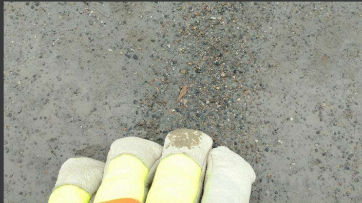
Removing Water From Surface Is Critical!
