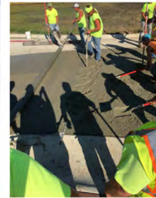
Figure 16- Using a portable vibrator and the roller screed for concrete placement
