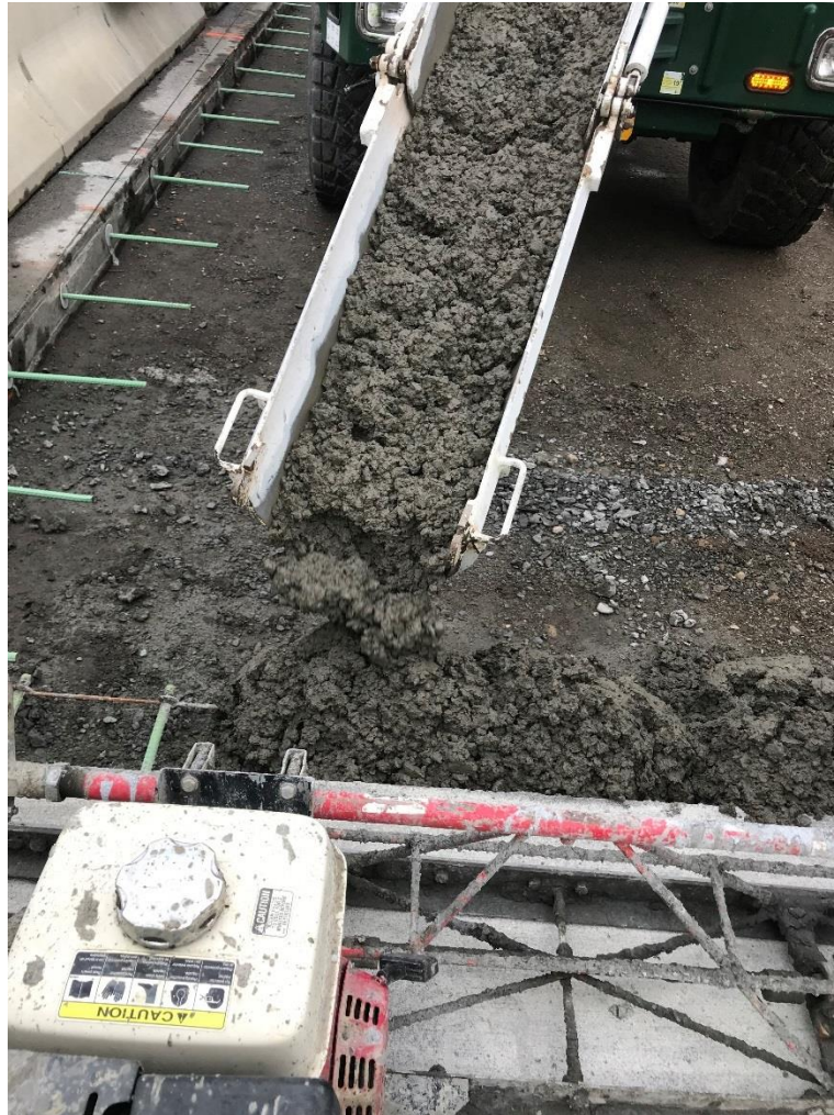
Figure 10 – PEM being placed
