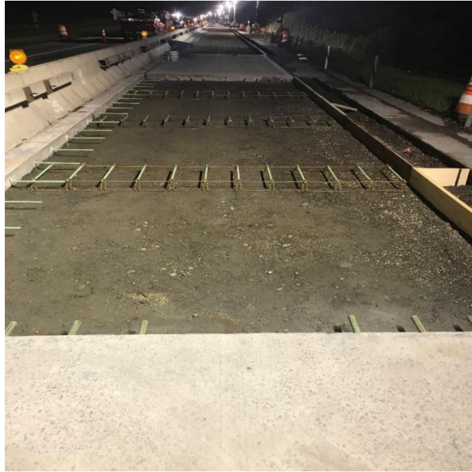
Figure 6 – Form work for new slabs
