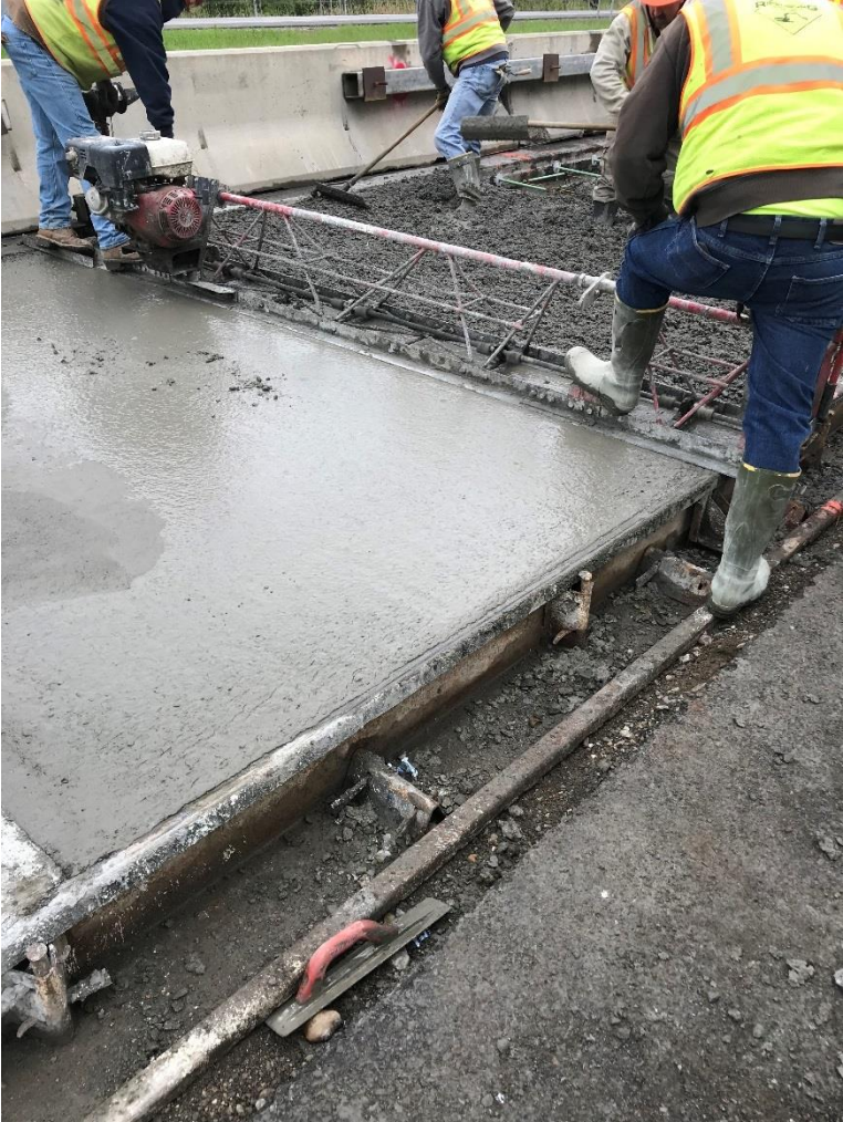
Figure 9 – PEM being placed
