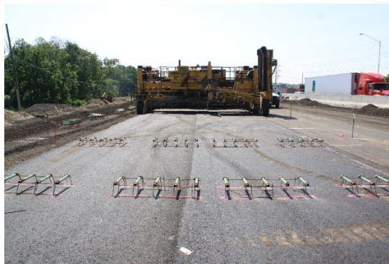
LOAD TRANSFER DOWEL BAR LAYOUT FOR NEW PAVEMENT
