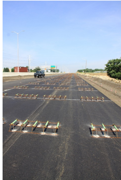
LOAD TRANSFER DOWEL BAR LAYOUT FOR NEW PAVEMENT
