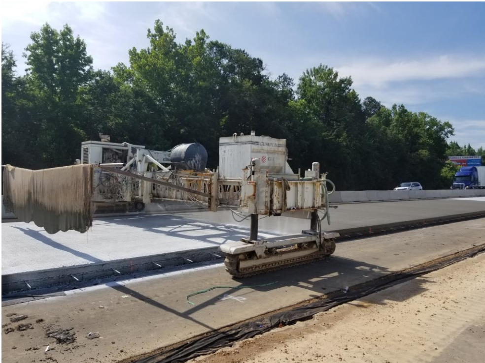
Figure 10: Application of curing compound.
