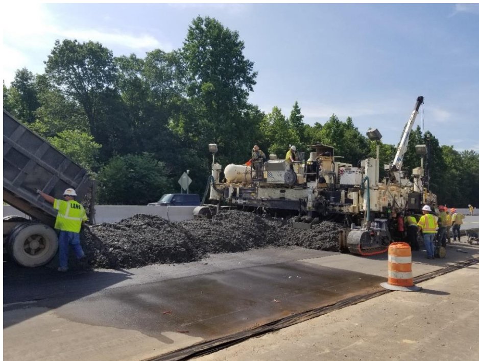
Figure 7: Concrete placed onto asphalt interlayer prior to entering paver.
