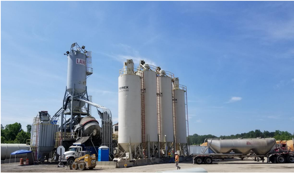
Figure 6: On-site batch plant at I-85 Widening in Rowan County, NC.
