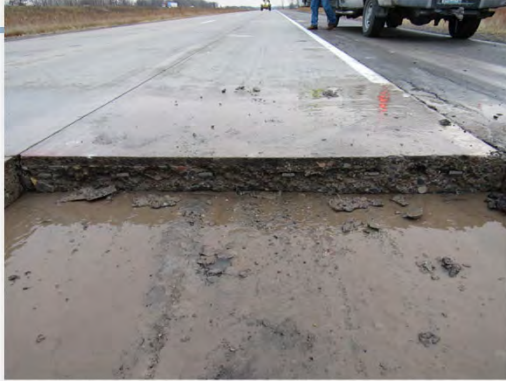
Cell 614, 12'L x 6'W panel replacement (shows plate dowels on basket).
