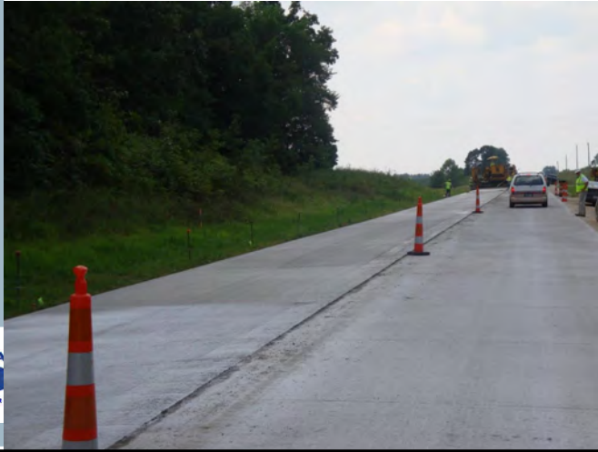
Local Traffic - one-way thru project
