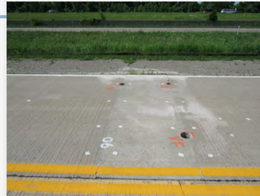
Cell 38, CoVex plate dowels in repair. 6+ dowels successful.
