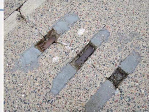
Cell 305 , Retrofit plate dowels in 5" UBOL
