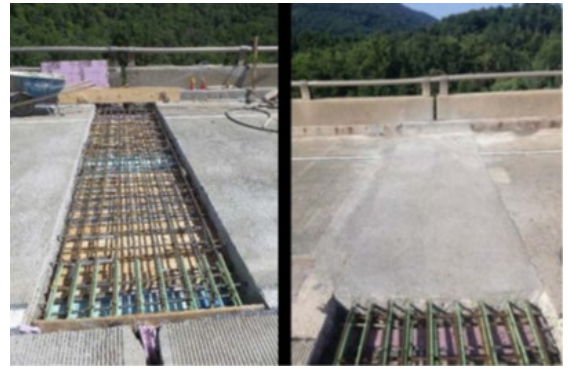
Concrete being placed on Dunlap Creek Bridge
