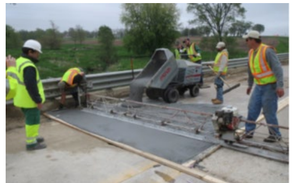
Workers pouring UHPC on a bridge deck
