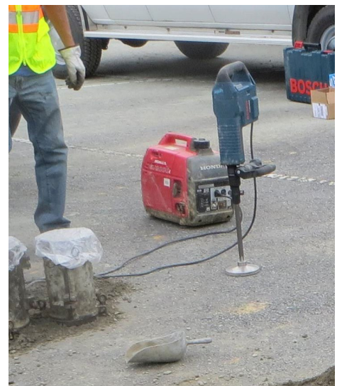
Vibrating hammer to prepare RCC cylinders
