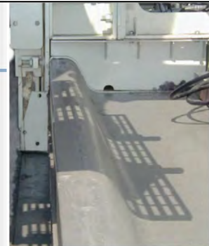
Figure 13. Slipform pavement with integral curb.
