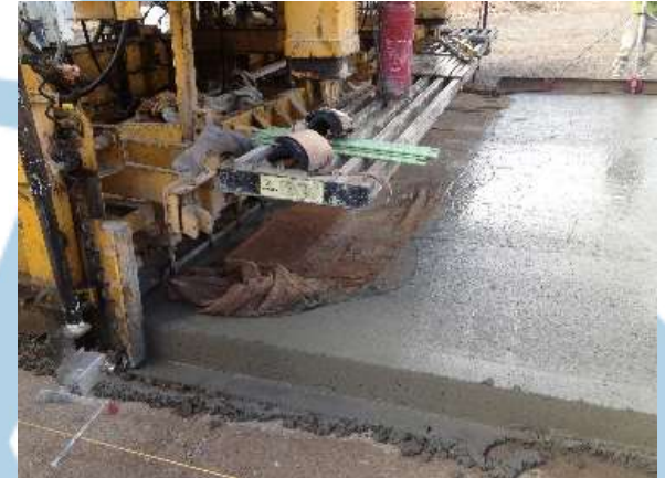
Placement of Nano Engineered Concrete
