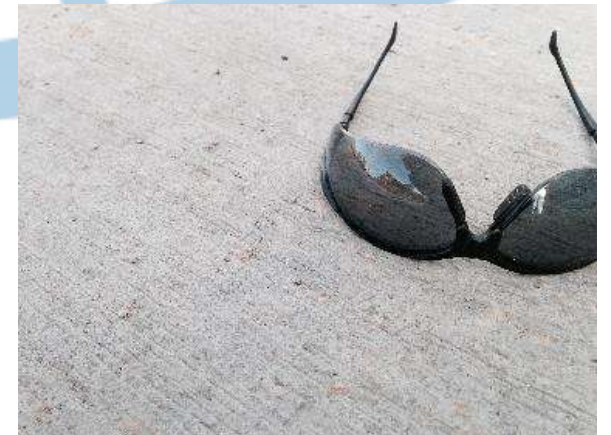
6 Years Later No Surface Defects / Cracking
