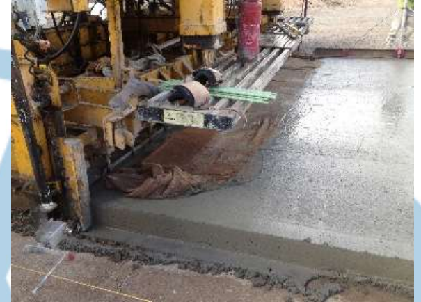
Placement of Nano Engineered Concrete
