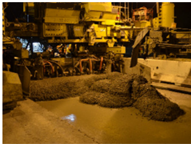
b. Top lift concrete in front of paver.
