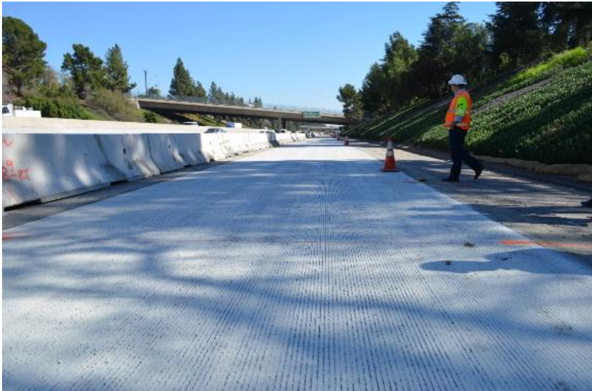
© Applied Pavement Technology
