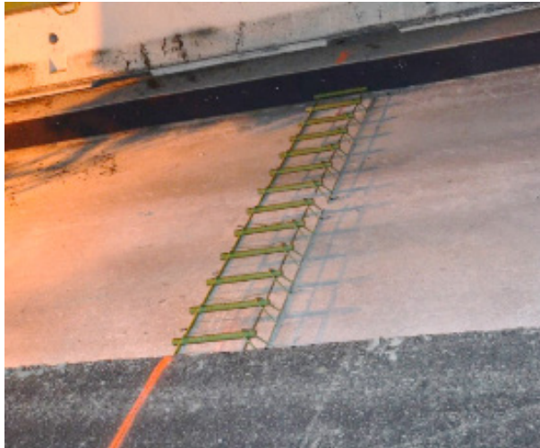
a. Dowel bars and basket anchors (and fiberboard).
