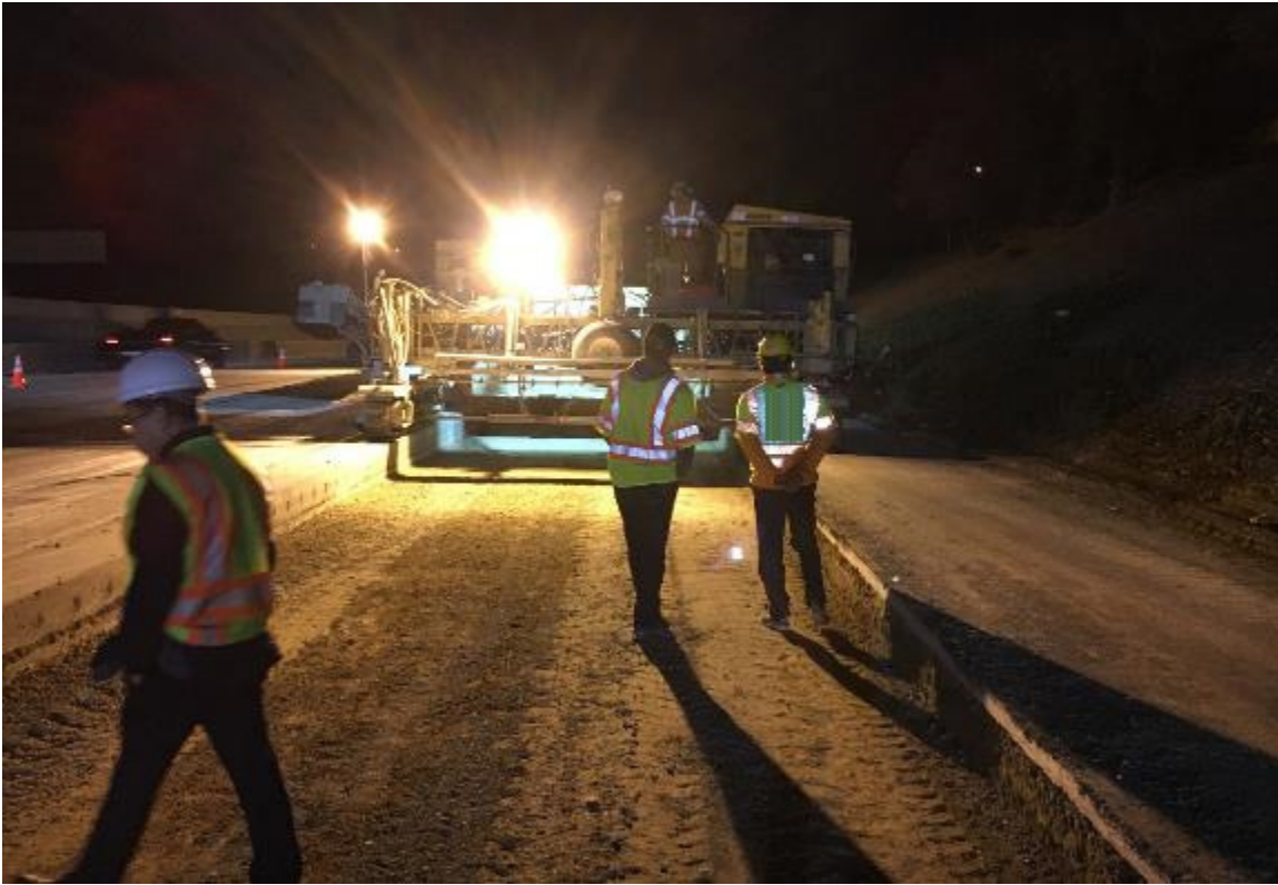
© Applied Pavement Technology
