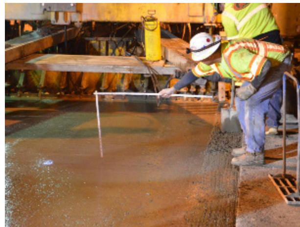
d. Close-up of bottom lift after paver.
