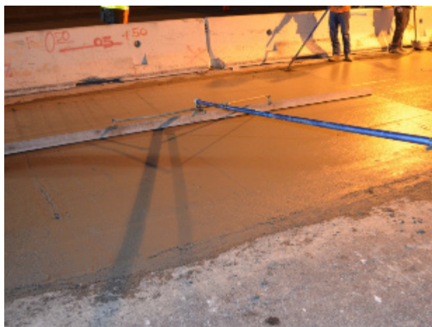
c. Bull floating operation on top lift.
