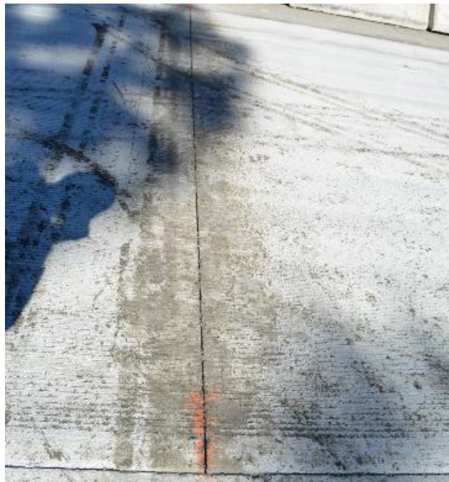
Figure 11. Transverse joint on new two-lift concrete pavement.
