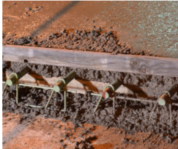
b. Close-up of dowel bar and basket at header.
