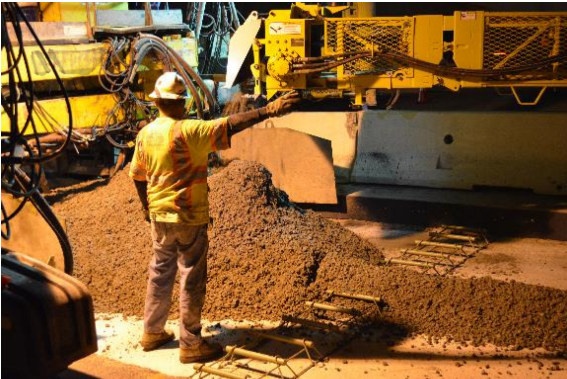
© Applied Pavement Technology
