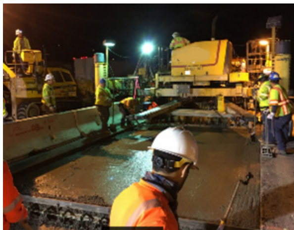
c. Bottom lift after going through paver.
