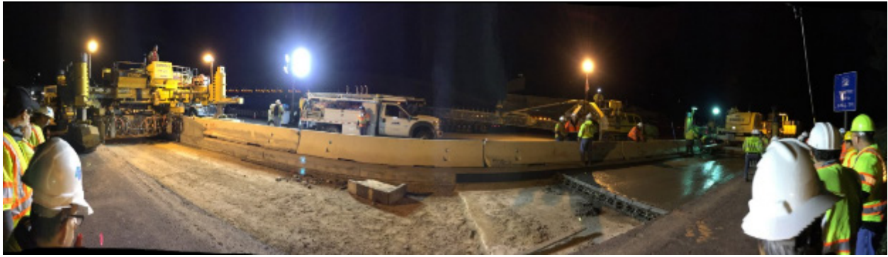
© Applied Pavement Technology
