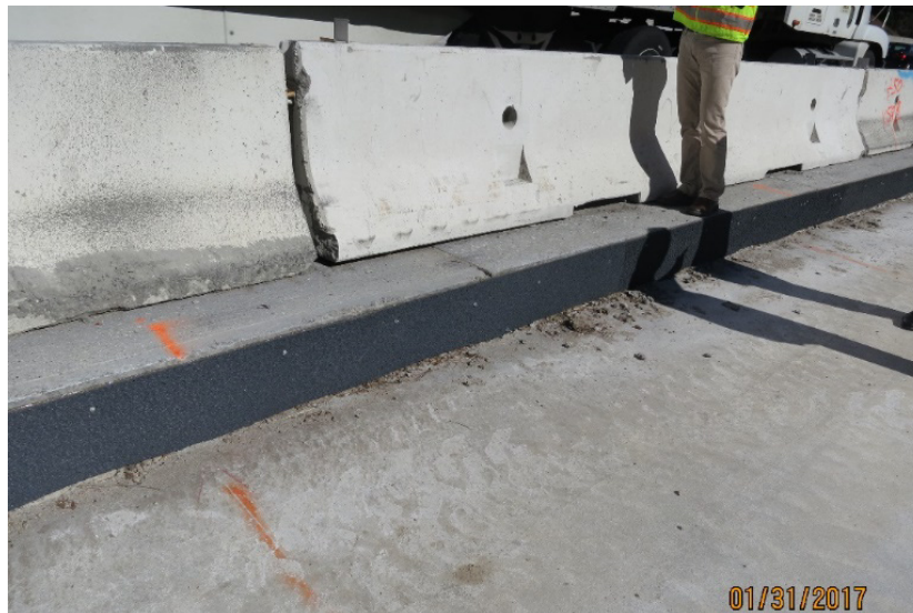
Figure 7. Fiberboard placed on adjacent pavement prior to paving two-lift section.
