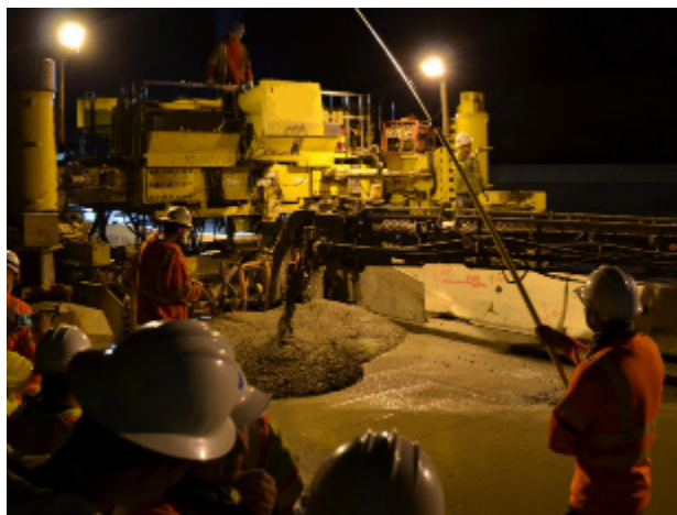
a. Delivery of top lift.
