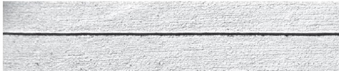
C. NO RAVELING - Sawed later in window
