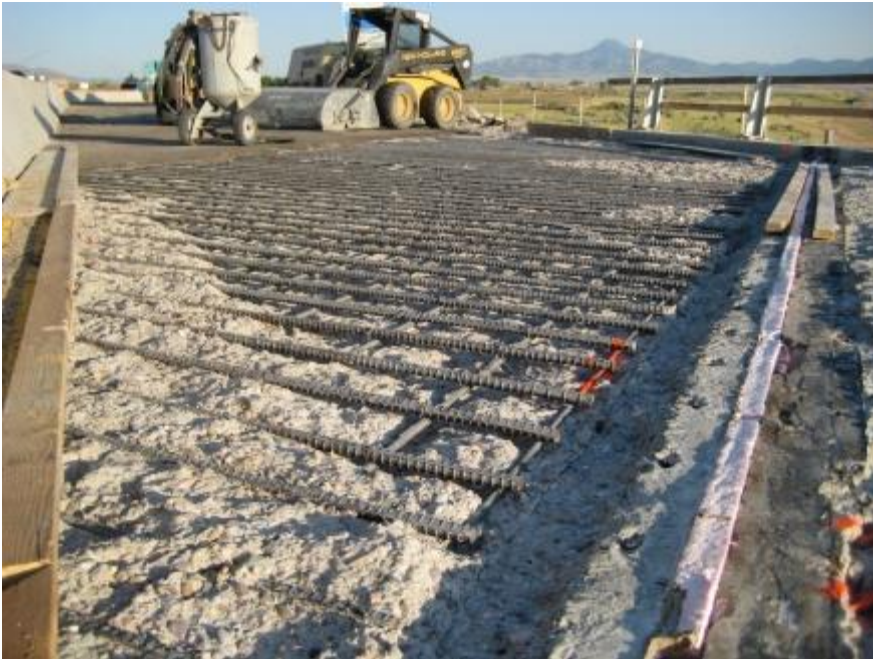
Deck repair/rehabilitation
