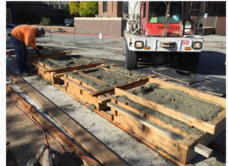
Casting the specimens
