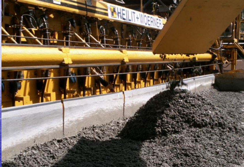
Paver for top lift
