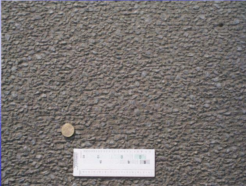
Surface after brushing
