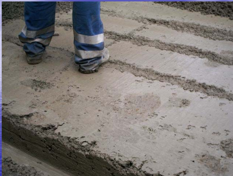
Stiff concrete for bottom lift
