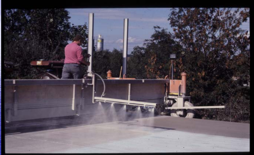
Curing compound on top of retarder
