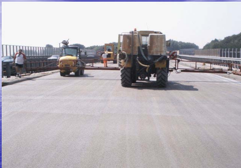
Curing (immediately!) after brushing
