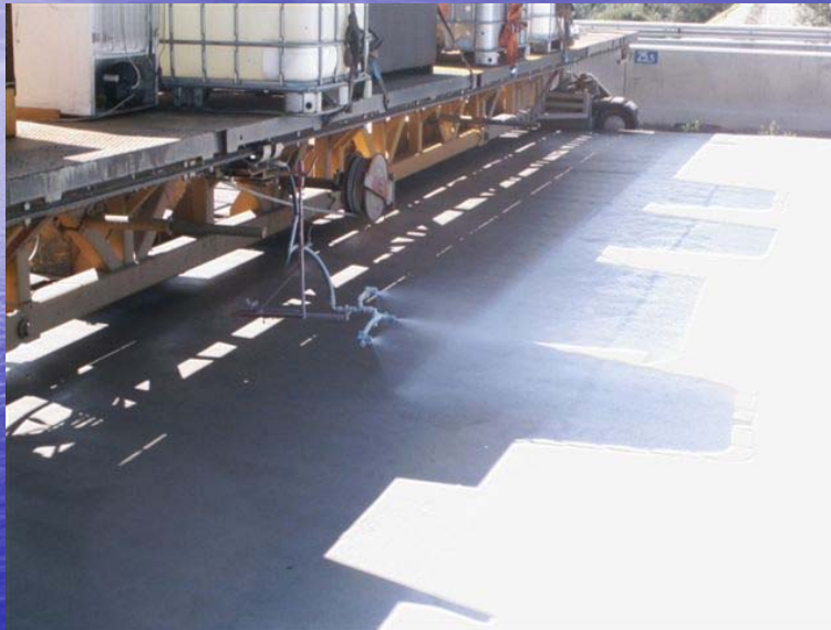
Spraying the combined (retarding and curing) compound
