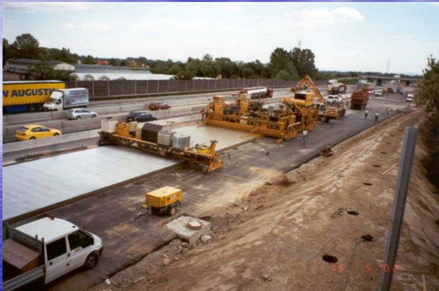
Paving train from behind
