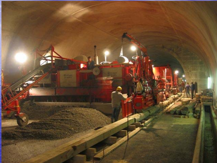
Paving in a tunnel
