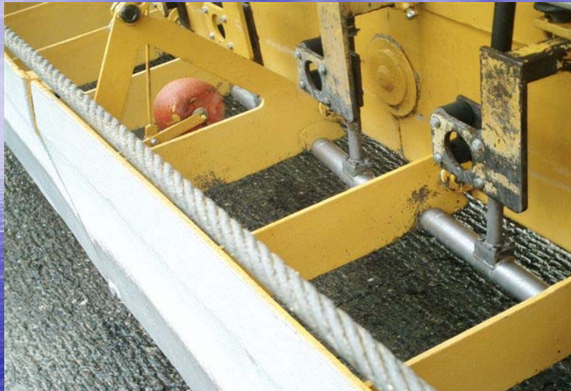
T-shaped vibrators (instead of pokers)
