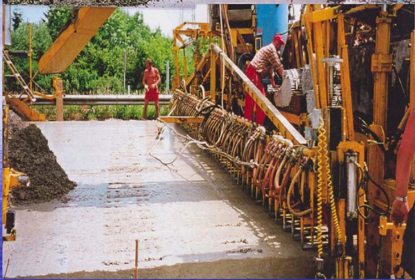
Bottom lift compacted, dowels inserted
