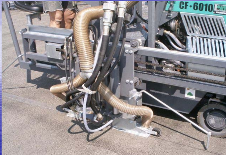
Sawing the joints
