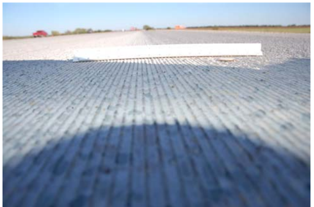
Figure 9: Surface E – Conventional Diamond Grinding (photo/test after grinding).
