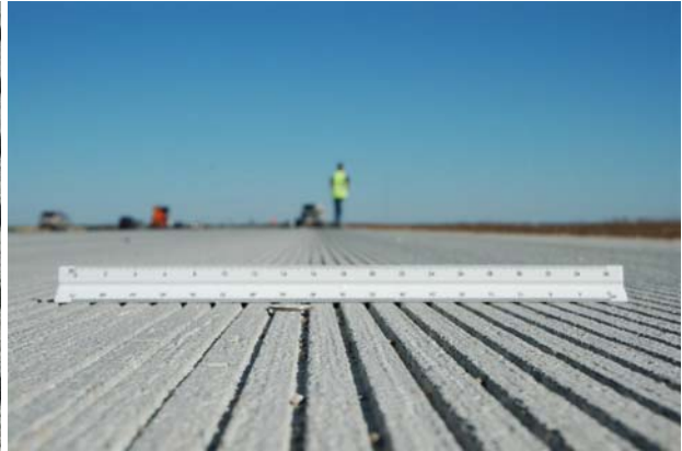
Figure 4: Surface B – Longitudinal Grooving + Burlap Drag (photo/test after grooving).
