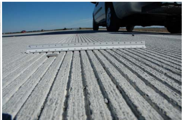
Figure 6: Surface C – Longitudinal Grooving + Turf Drag (photo/test after grooving).
