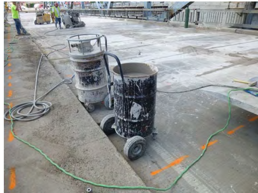
55 (Photo: Dwayne Stenlund, MnDOT)
