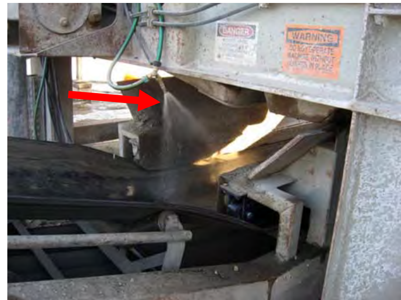
Photo: Dwayne Stenlund, MnDOT
