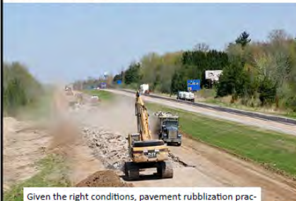
BMP 4. Multihead pavement breaker rubblization. Water mists not need this day.
