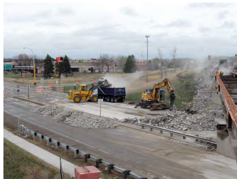
Photo: Dwayne Stenlund, MnDOT
