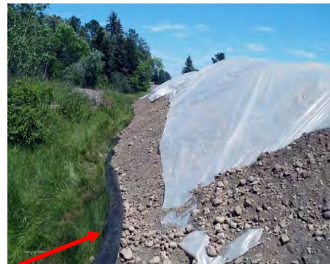
Plastic cover and perimeter berm
