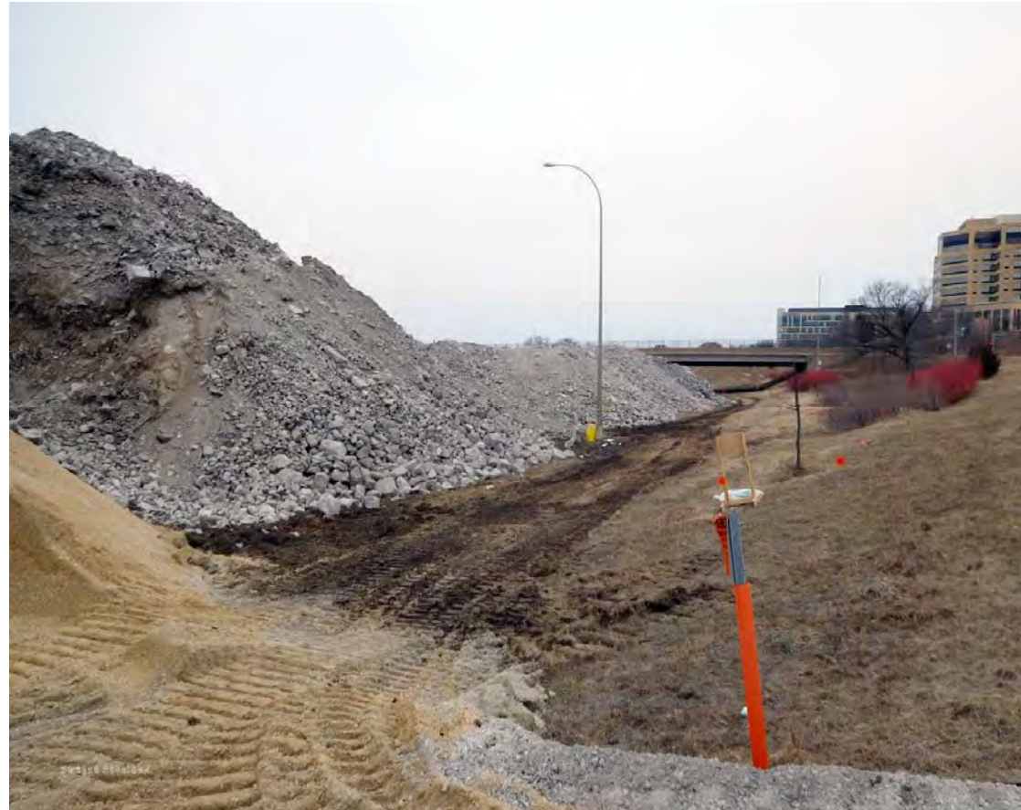
Stockpiles for crushing set inside roadway depression with inlets offline
