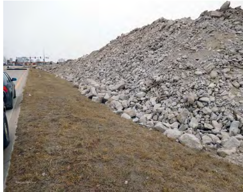
Photo: Dwayne Stenlund, MnDOT
