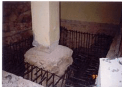
Fig. 3: Installing the main steel in footing
