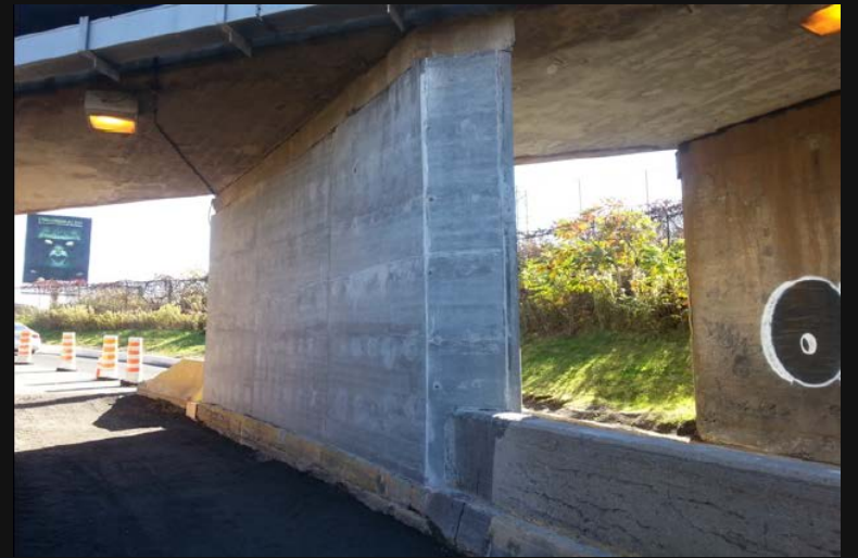
CN Rail Bridge Pier Jacketing, Montreal, QC
