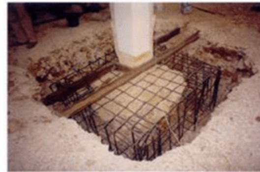
Fig.4: Completing the jacketing of footing
