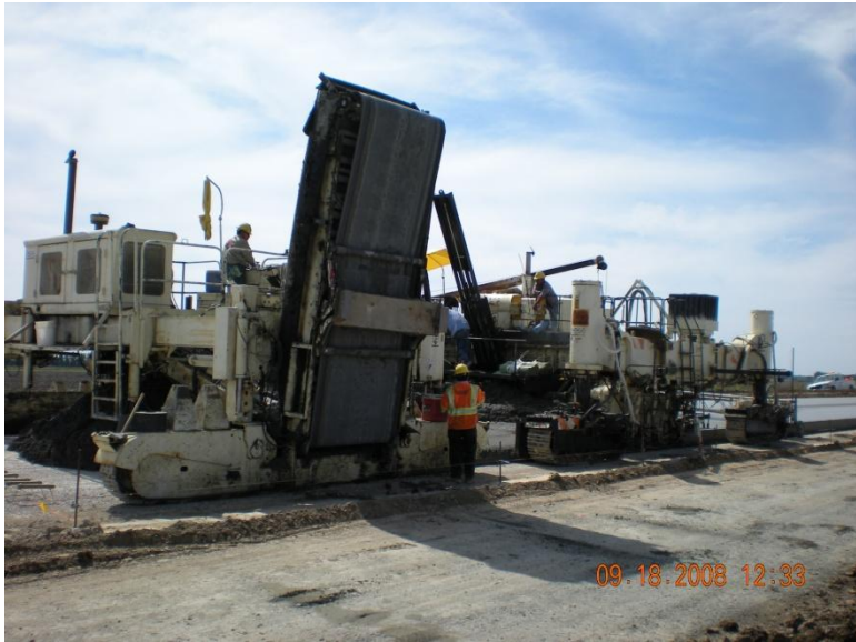
Figure 30 Bottom Lift Belt Placer/Spreader and Paver
