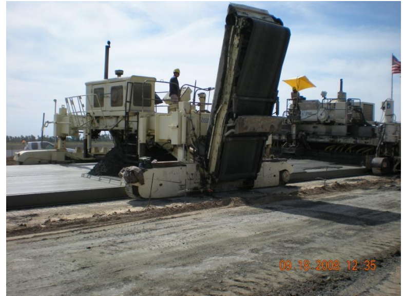
Figure 31 Top Lift Belt Placer/Spreader and Paver
