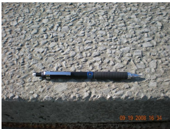
Figure 37 Exposed Aggregate Surface
