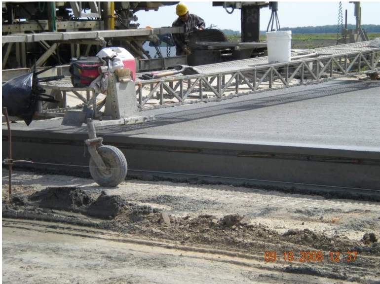
Figure 32 Initial Burlap Drag Following Top Lift Paver
