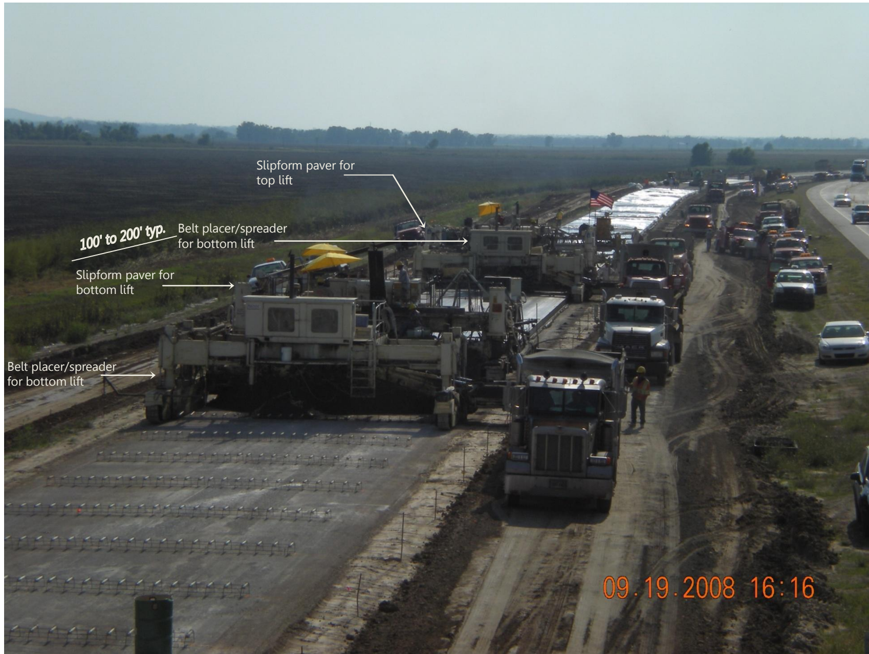
Figure 29 I-70 Two-Lift Paving Equipment Train
