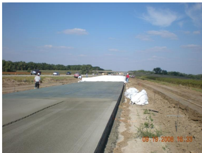
Figure 34 Removing Polyethylene Sheeting in 100' Segments
