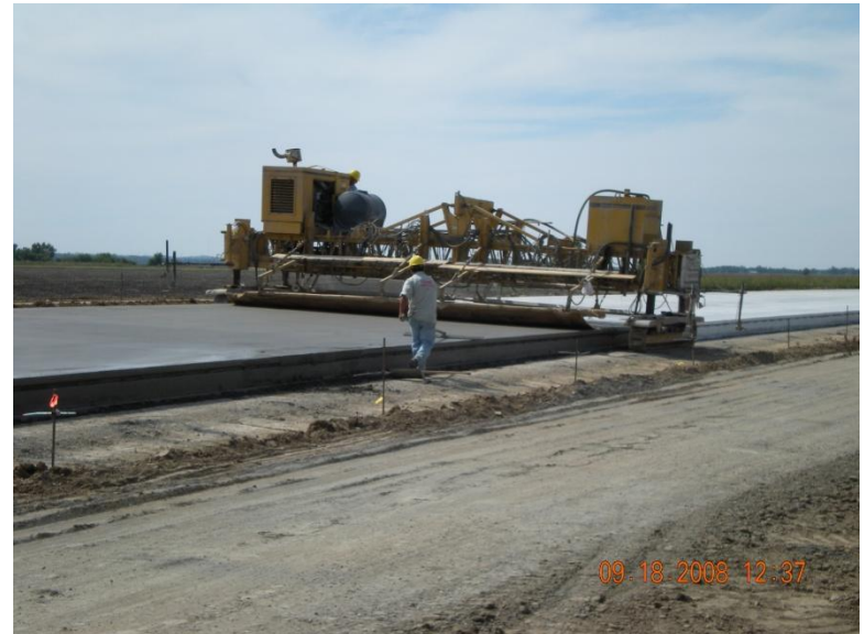
Figure 33 Texture/Cure Machine Following Final Finishing
