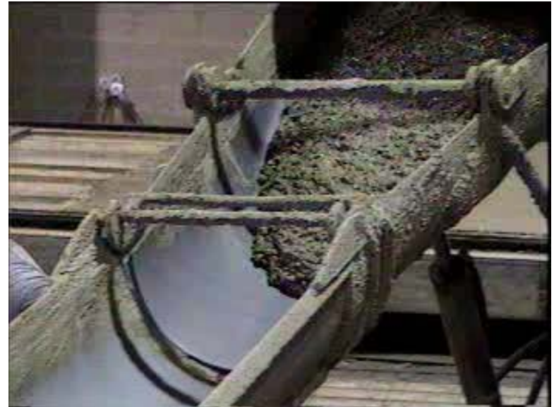
Flowing into double T beam forms ACI 237 ETS Report
