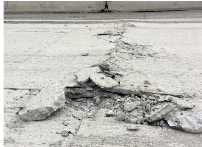
Blowup in Jointed Concrete Pavement
