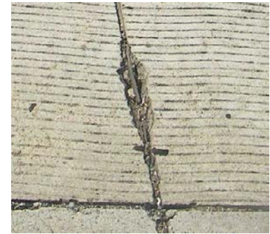
Incompressible joint damage
