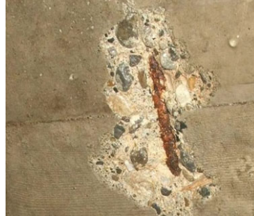
Chloride penetration
