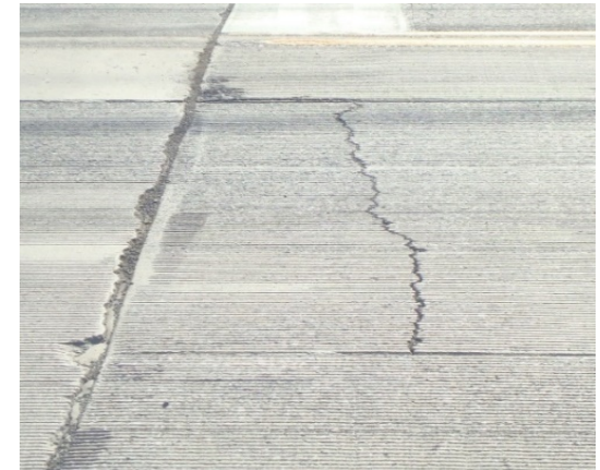
Reflective Cracks
