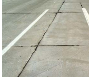
Early saw joint raveling
