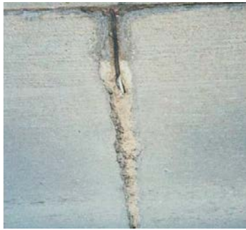
Saturated joint backer rod damage
