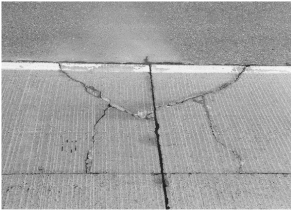
Corner Cracks
