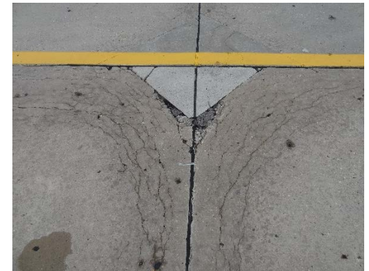
Staining Accompanying D-Cracking at Joints
