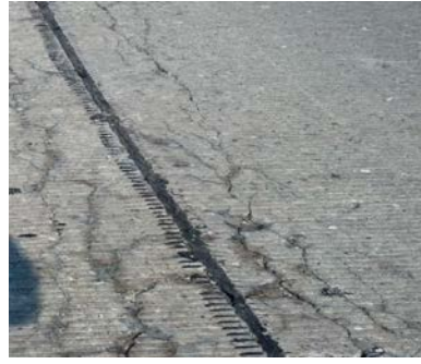
Saturated joint with unsound aggregate
