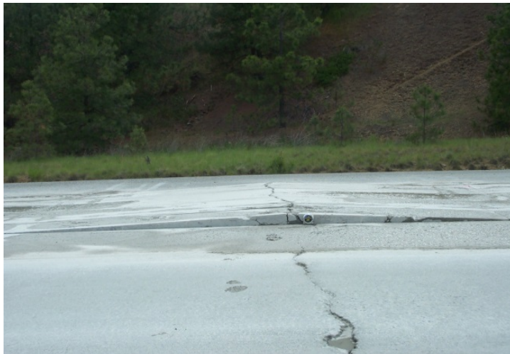
Blowup in Jointed Concrete Pavement
