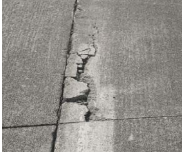
Deflection spalling from heavy vertical loads
