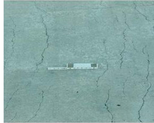
Plastic Shrinkage Cracking
