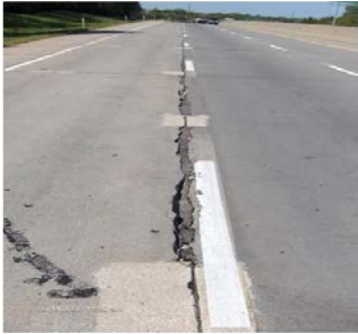
Freeze thaw damage
