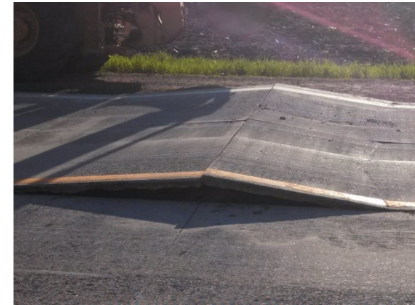
Blowup Crack
