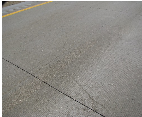
Reflective Crack
