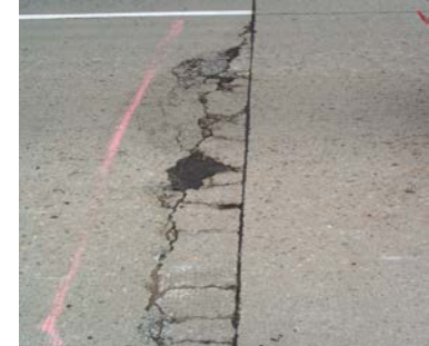
Dowel bar misalignment
