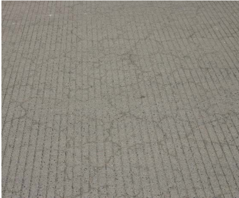
Map Cracking
