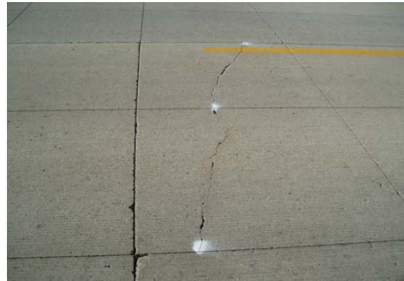
Longitudinal Cracks Transverse Crack
