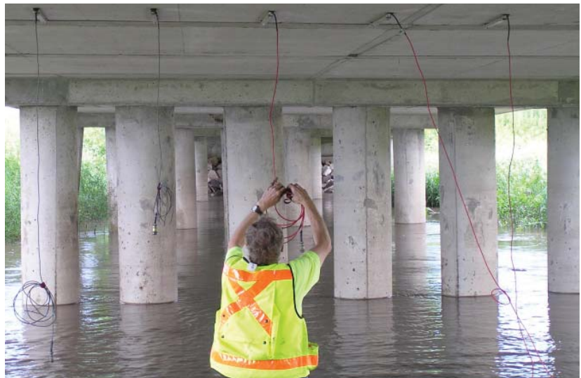
Bridge being instrumented
