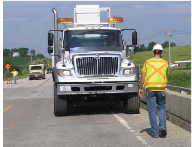
Positioning of load truck for static load test
