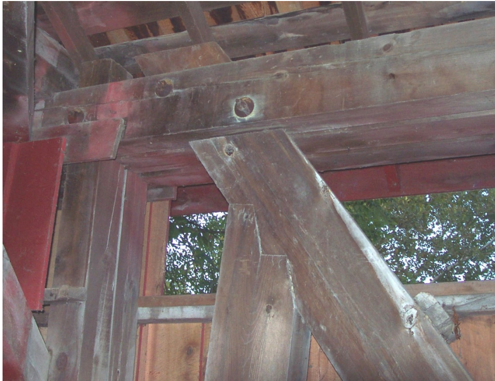
Figure 10. Cataract Bridge, Owen Co, IN (detail). The zigzag notching of post and brace in the outermost panels is characteristic of the Smith Bridge Company. Photo: J.A. Barker Engineering
