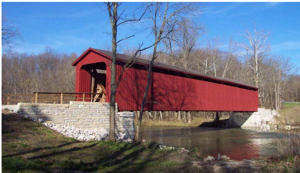
Figure 1. Cataract Covered Bridge, an 1876 Smith truss structure. 2006 (post-rehabilitation) photo by the author.
