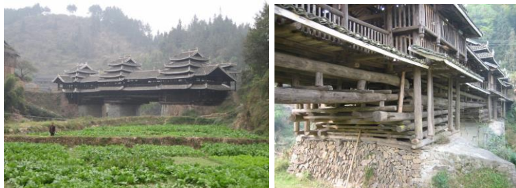
Cantilevered ‘wind and rain’ Batuan Bridge, Sanjiang district, Guangxi Province. Photographs by Ronald G. Knapp, 2006
