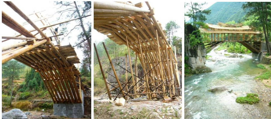
Construction of the Tongle Bridge, Taishun, Zhejiang, 2004-2006 Photographs by Xue Yichuan
