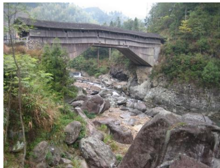
The Yuanfeng Bridge in Shouning County, Fujian has a span of 37.6 meters. Photograph by Ronald G. Knapp, 2006
