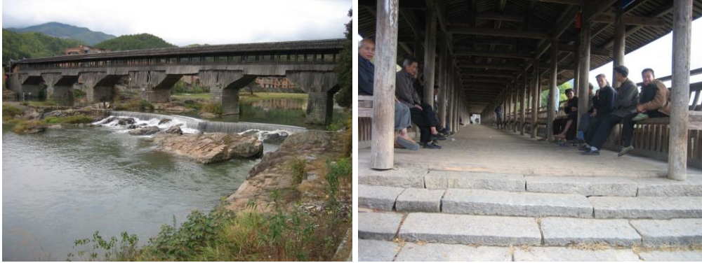
Wan'an Bridge, Pingnan County, Fujian Photograph by Ronald G. Knapp, 2006
