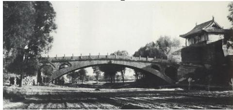
Anji Bridge, Hebei, 1933. Source: Liang Sicheng, 1982: 240
