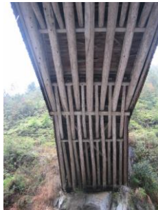
Underside of Santiao Bridge, Taishun County, Zhejiang Province.
