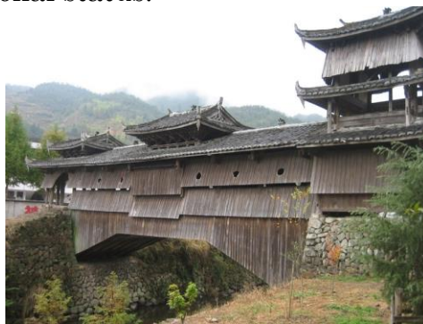
The Rulong or "Like a Dragon" Bridge was built in the later part of the Ming dynasty in 1625. Photograph by Ronald G. Knapp, 2006
