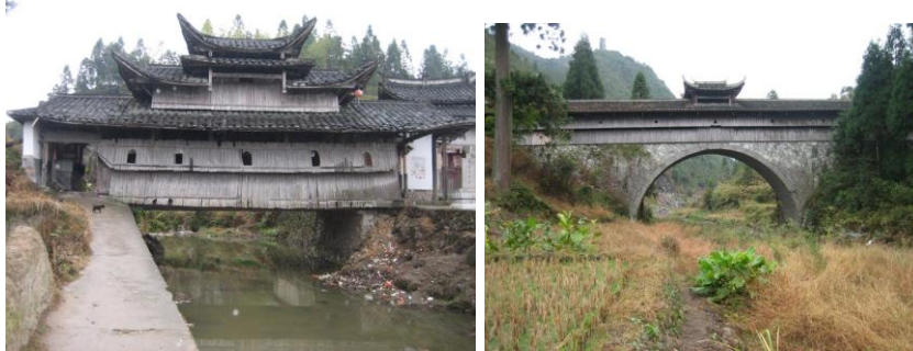
Left: Yingjie Temple Bridge, Qingyuan County, Zhejiang Right: Buchan Bridge, Qingyuan County, Zhejiang Photographs by Ronald G. Knapp, 2006
