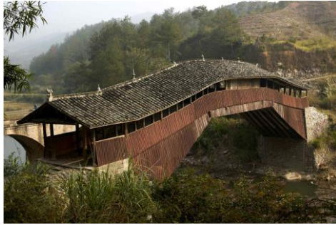
Xianju Bridge, Taishun County, Zhejiang, first built in 1483. , has a span of 35 meters, just 2 meters shorter than that of the Anji Bridge and it rises higher above the water than the Qingming shanghe tu rainbow bridge.
