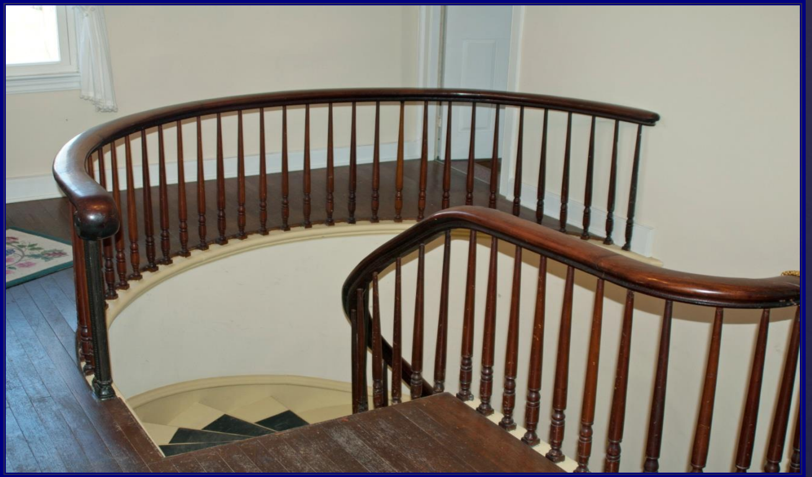
Upstairs View of Staircase
