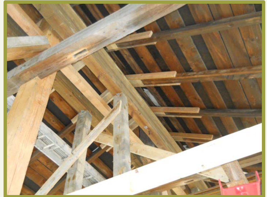
Sistered Roof Rafters
