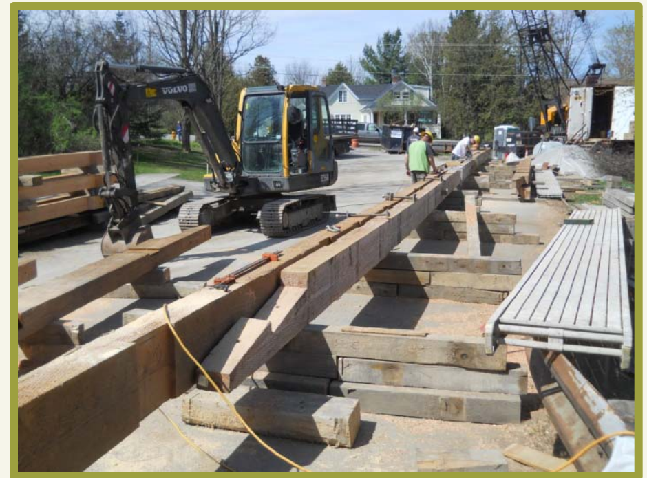
New Bottom Chord
