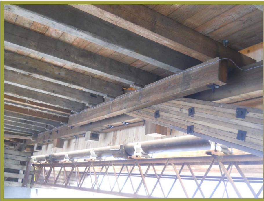
Typical Floor Framing at Arch Locations
