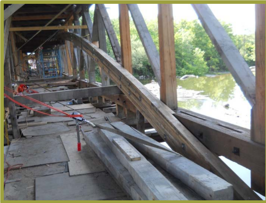
Rebuilt East End of North Arch
