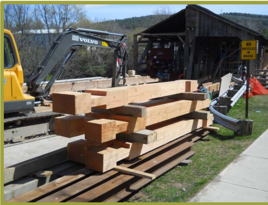
New Truss Verticals
