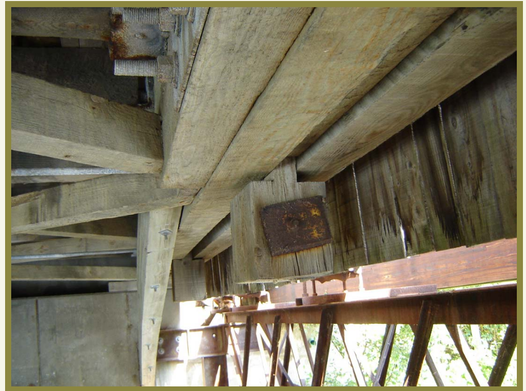
Undersized Verticals At Notch
