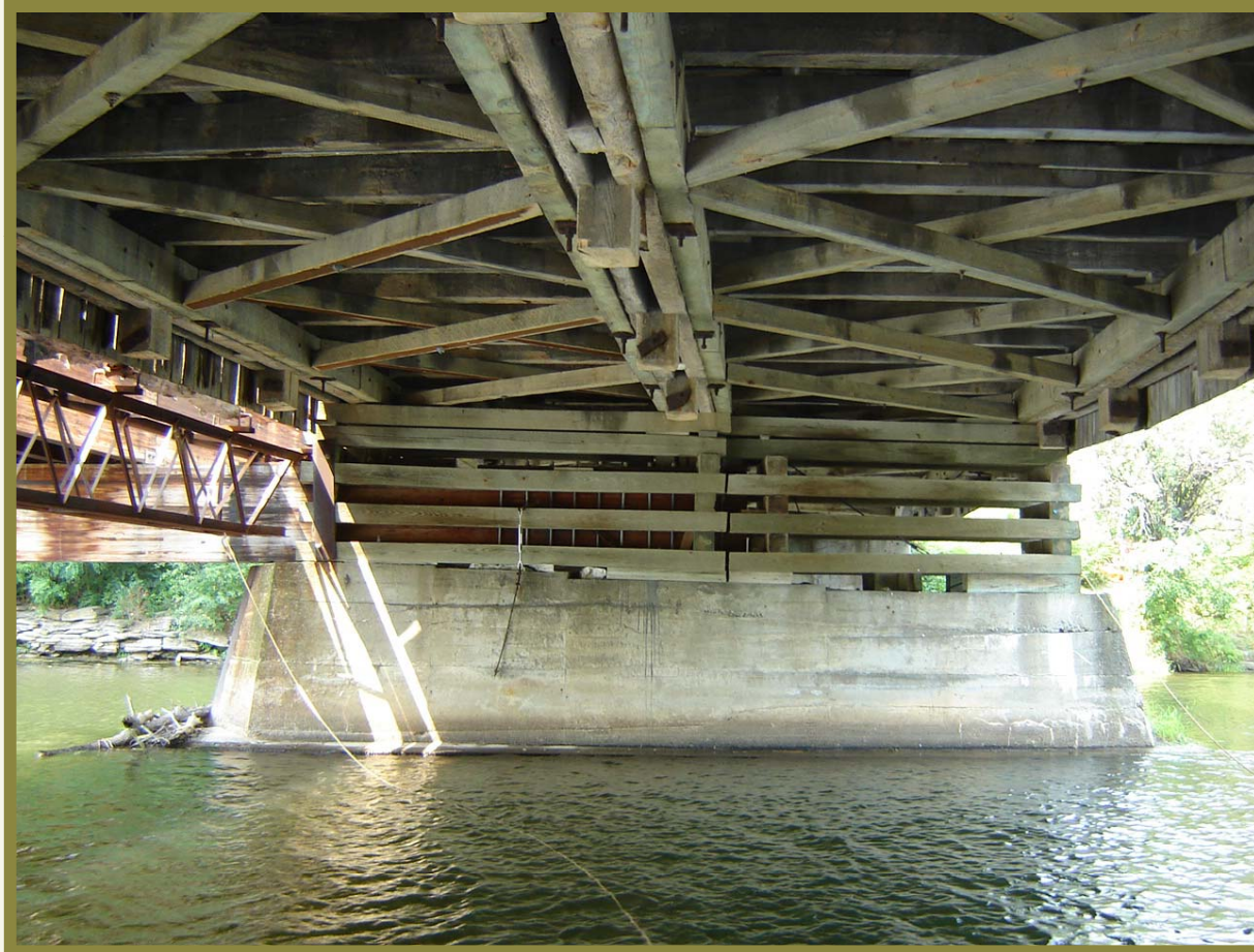
Bridge East Pier & Floor Framing
