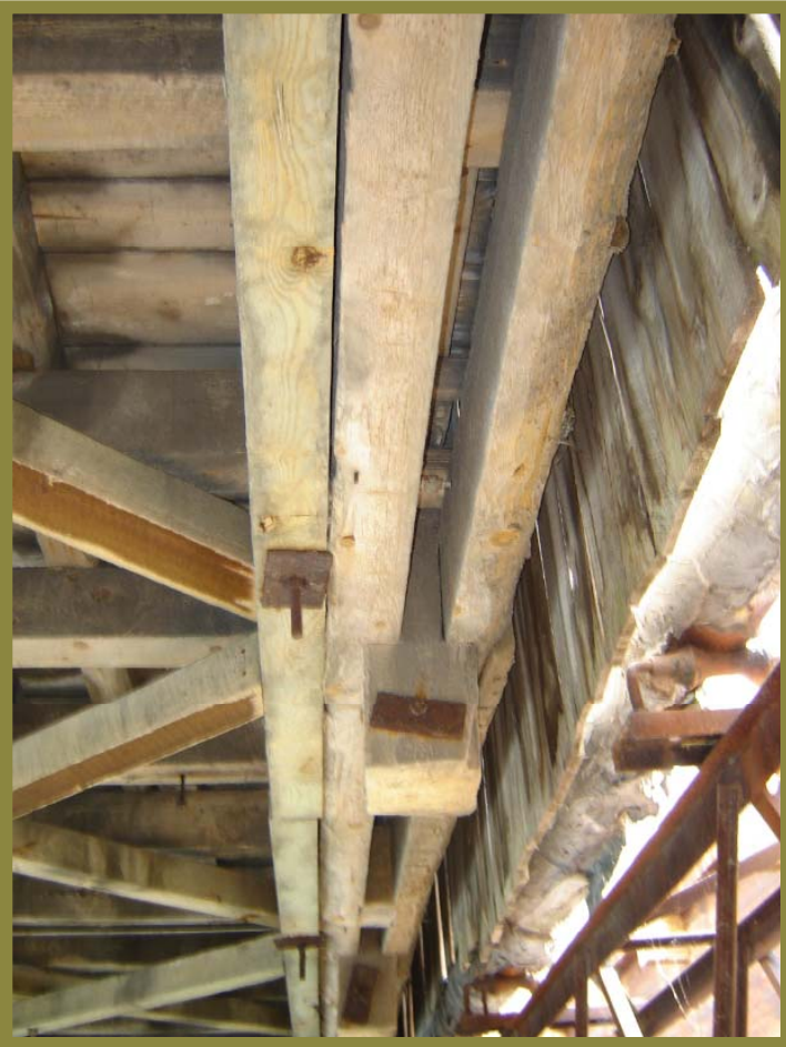
Undersized Verticals At Notch
