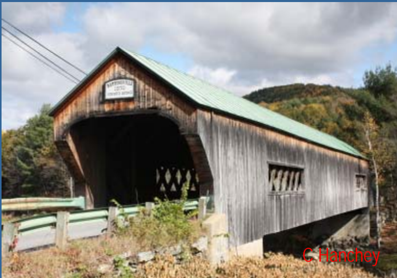
Old Bartonsville Bridge – October 2009
