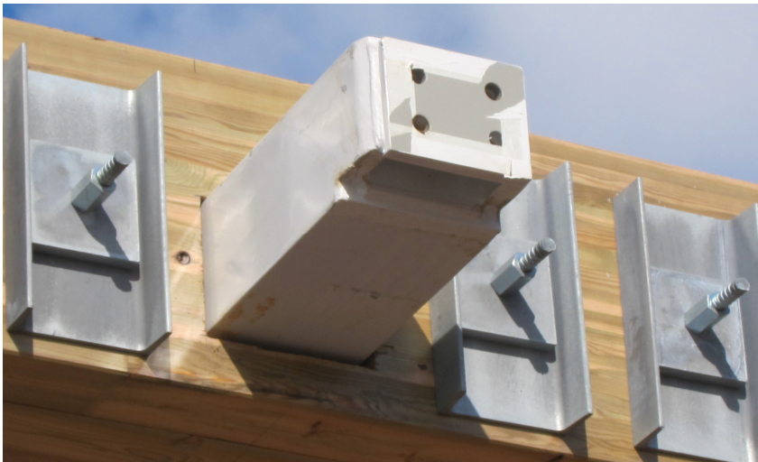
Fig. 12 Picture of crossbeam and bar anchor plates
