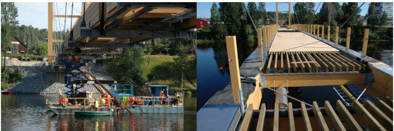
Figure 15: Finishing construction work after pulling out all the bridge decks.
