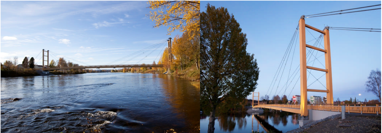
Fig. 1: Views of the final result of “The Älvsbacka Bridge”
