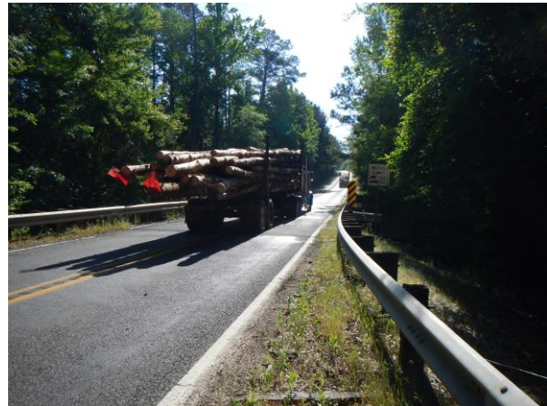
Fig. 13 View of logging trucks traversing bridge
