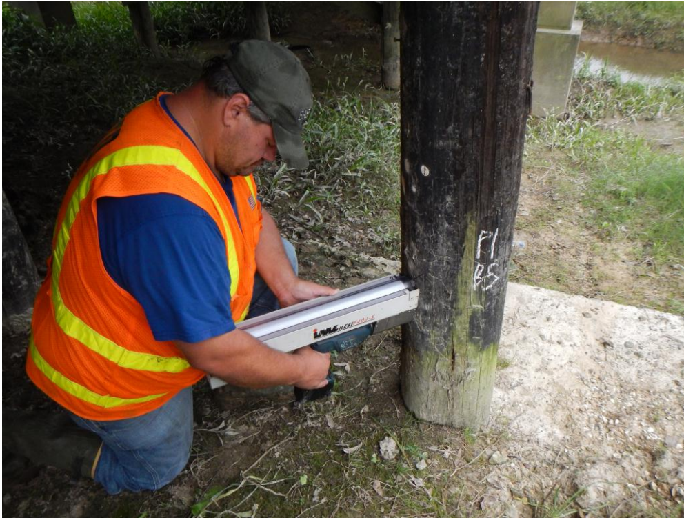
Fig. 6 Resistance Microdrilling to assess condition of pile suspected of being hollow
