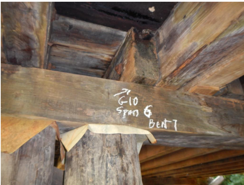
Fig. 7 Labeling of girder locations for reference
