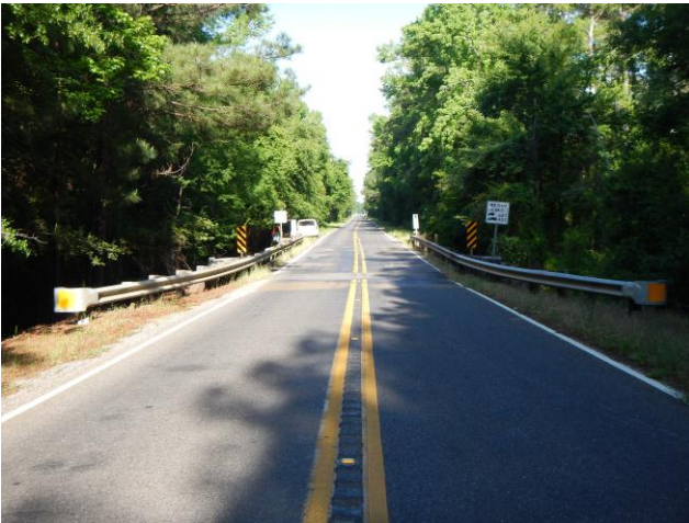
Fig. 8 View of Approach to Bridge 08-4
