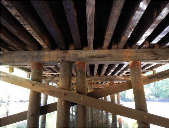
Fig. 16 Stringers supporting timber deck
