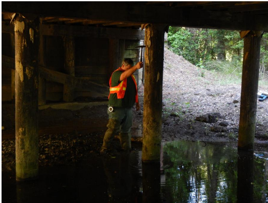
Fig. 3 Inspector using hammer to assess condition of pile from sound
