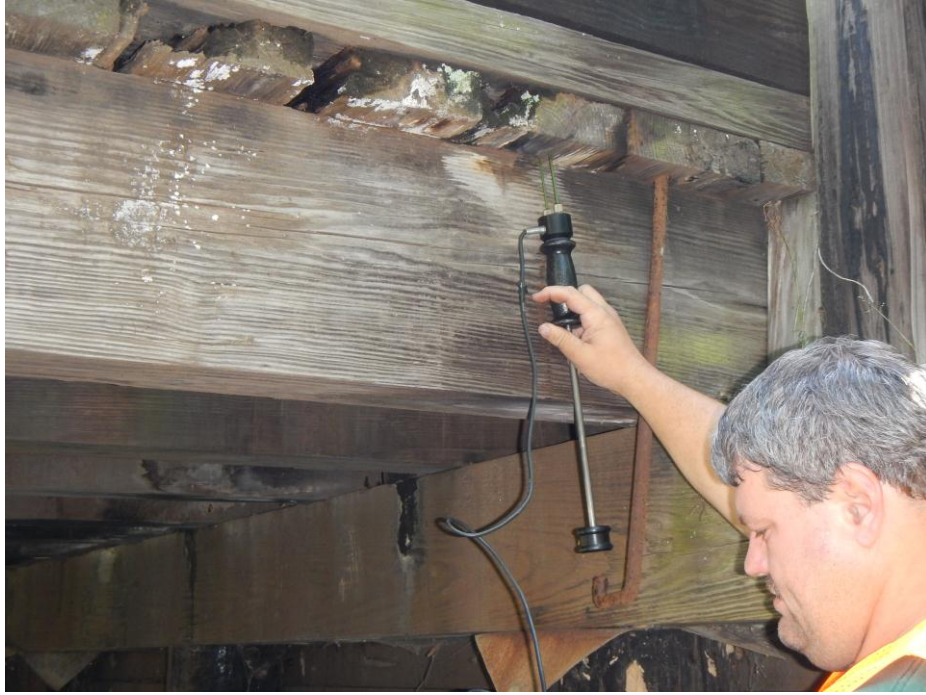
Fig. 4 Determining moisture content of wood deck with moisture meter
