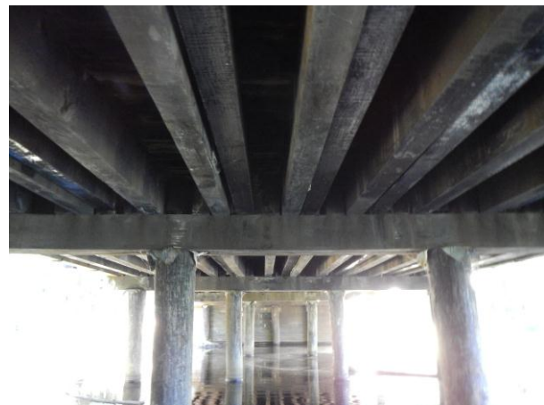
Fig. 11 Stringers supporting timber deck
