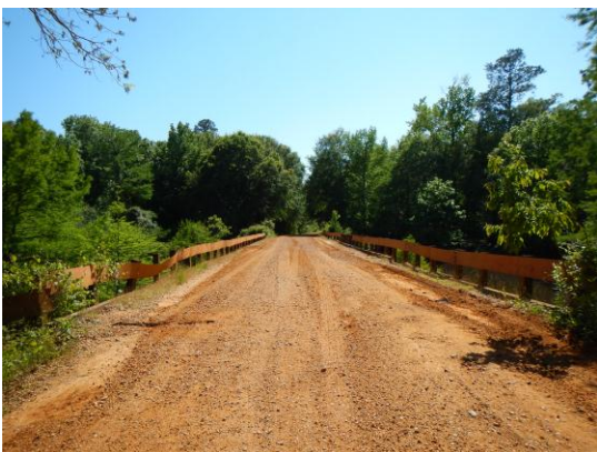
Fig. 14 View of Approach to Bridge 08-2
