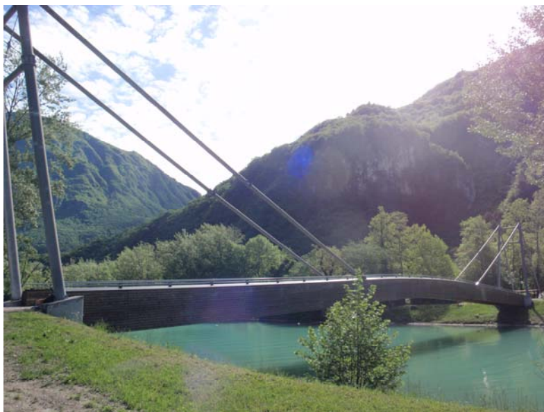
Fig. 2 Lateral view of the pedestrian timber bridge under study.
