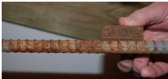
Fig. 21 Corroded tendon bar on a 17-year-old bridge
