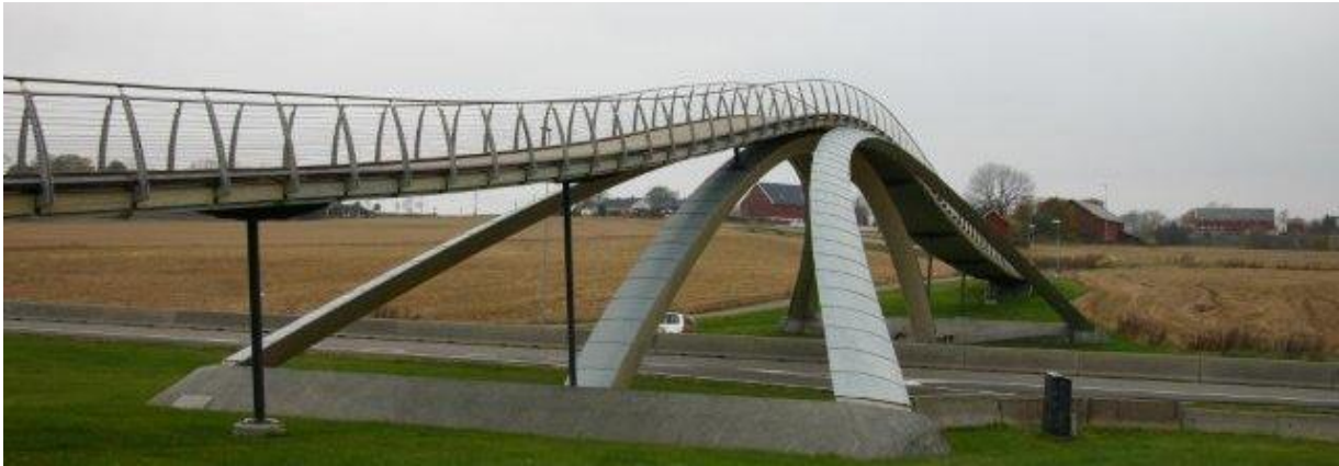
Fig. 14 The Leonardo da Vinci bridge also had fungus attack before it received structural protection to its upper face of the arcs. Constructed in 2005
