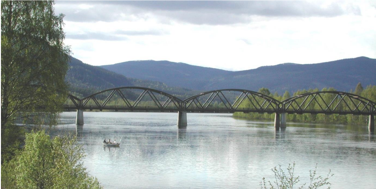
Fig. 1 Evenstad Bridge, constructed in 1996, five spans, dual carriageway, total length 180 m
