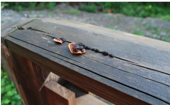
Fig. 13 Fungi is growing on a horizontal member. The photo is taken in 2009.
