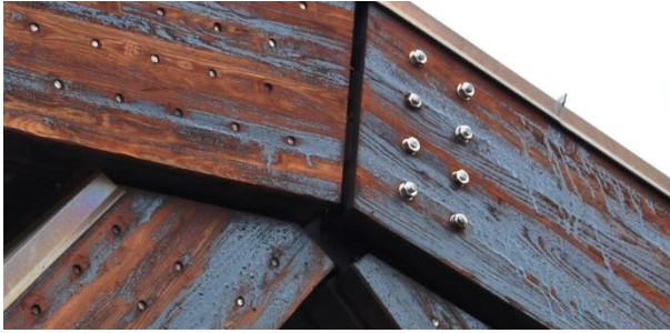
Fig. 20 Dowels fastened with nuts
