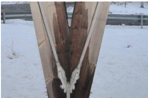
Fig. 6 A V-shaped column with stays.
