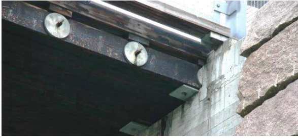
Fig. 11 The timber deck are in direct contact with the concrete
