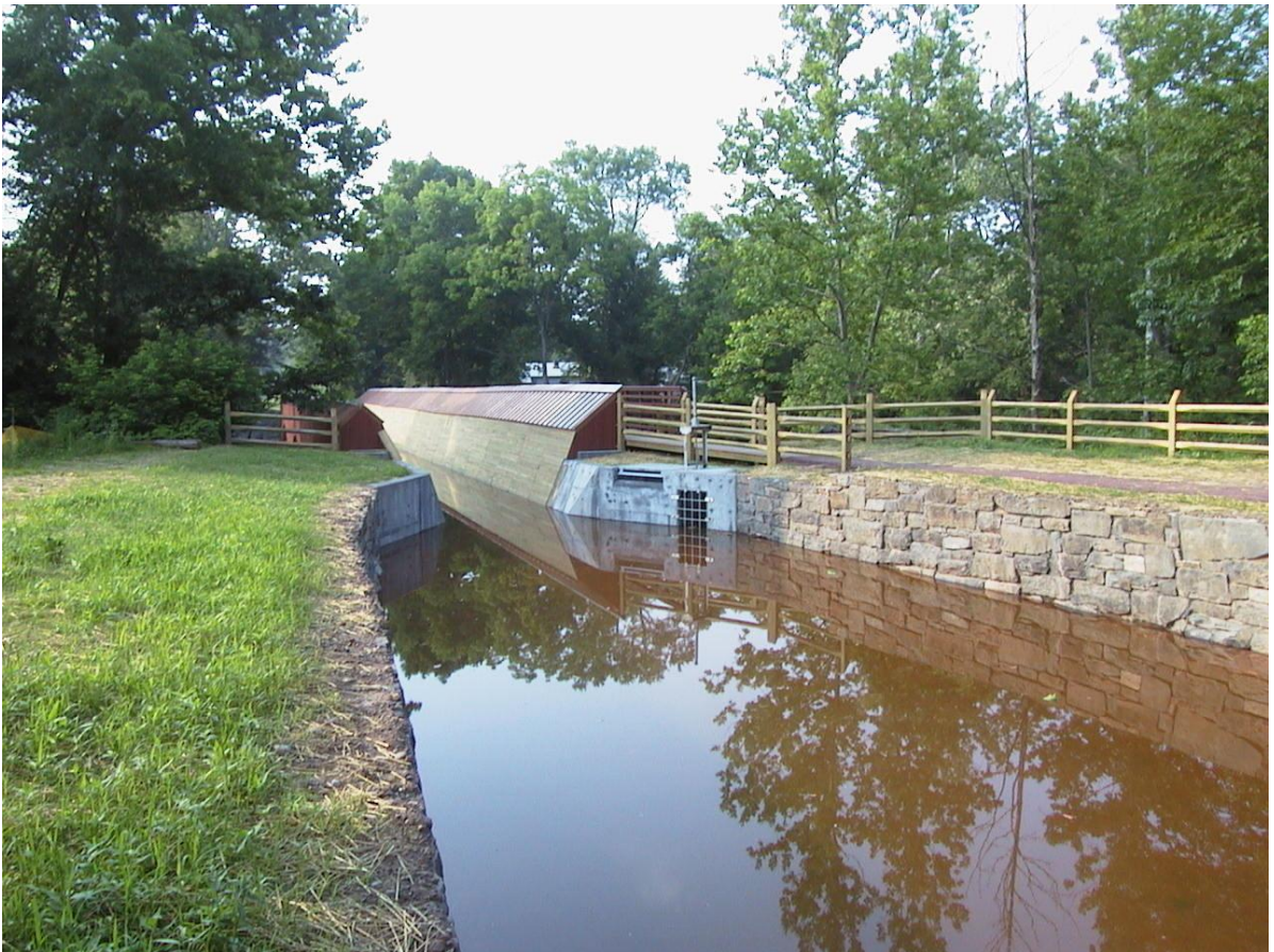
Figure 10 View north of the new Tohickon Aqueduct, partially watered
