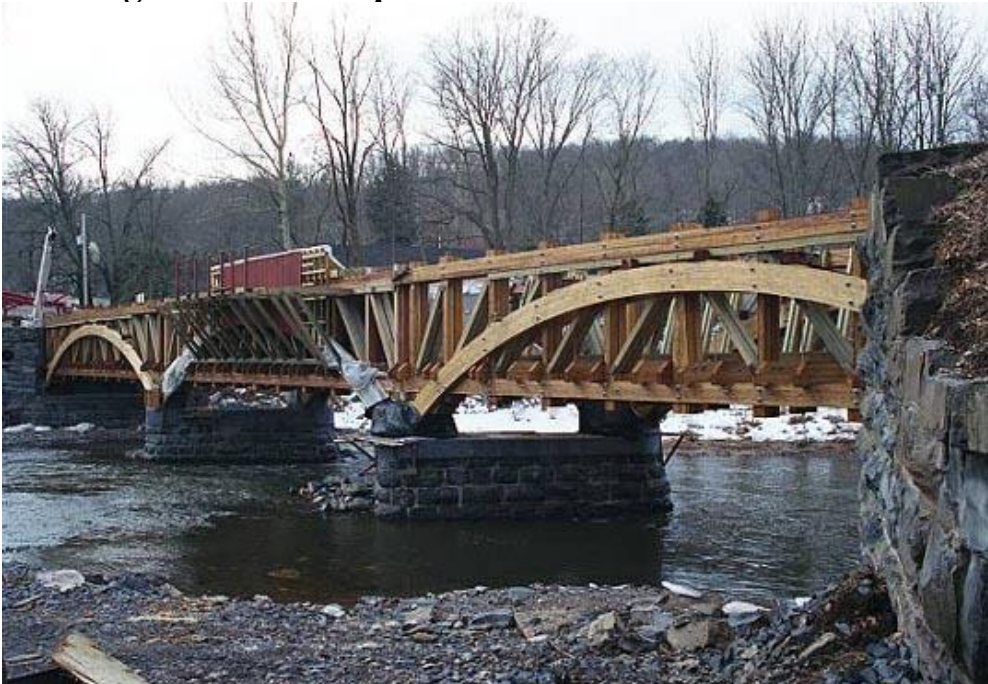
Fig.6: The eastern elevation of the Tohickon Aqueduct during construction
