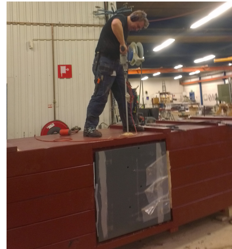
Fig. 10 Insertion of dowels in the arch
