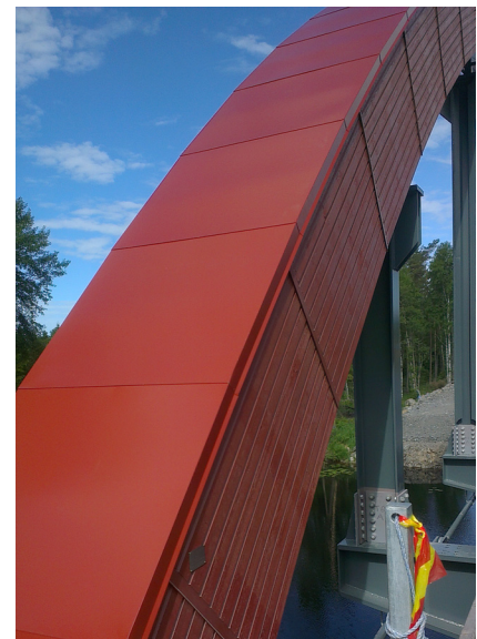
Fig. 9 Ventilated wood panel and steel sheeting to protect the glulam arches.
