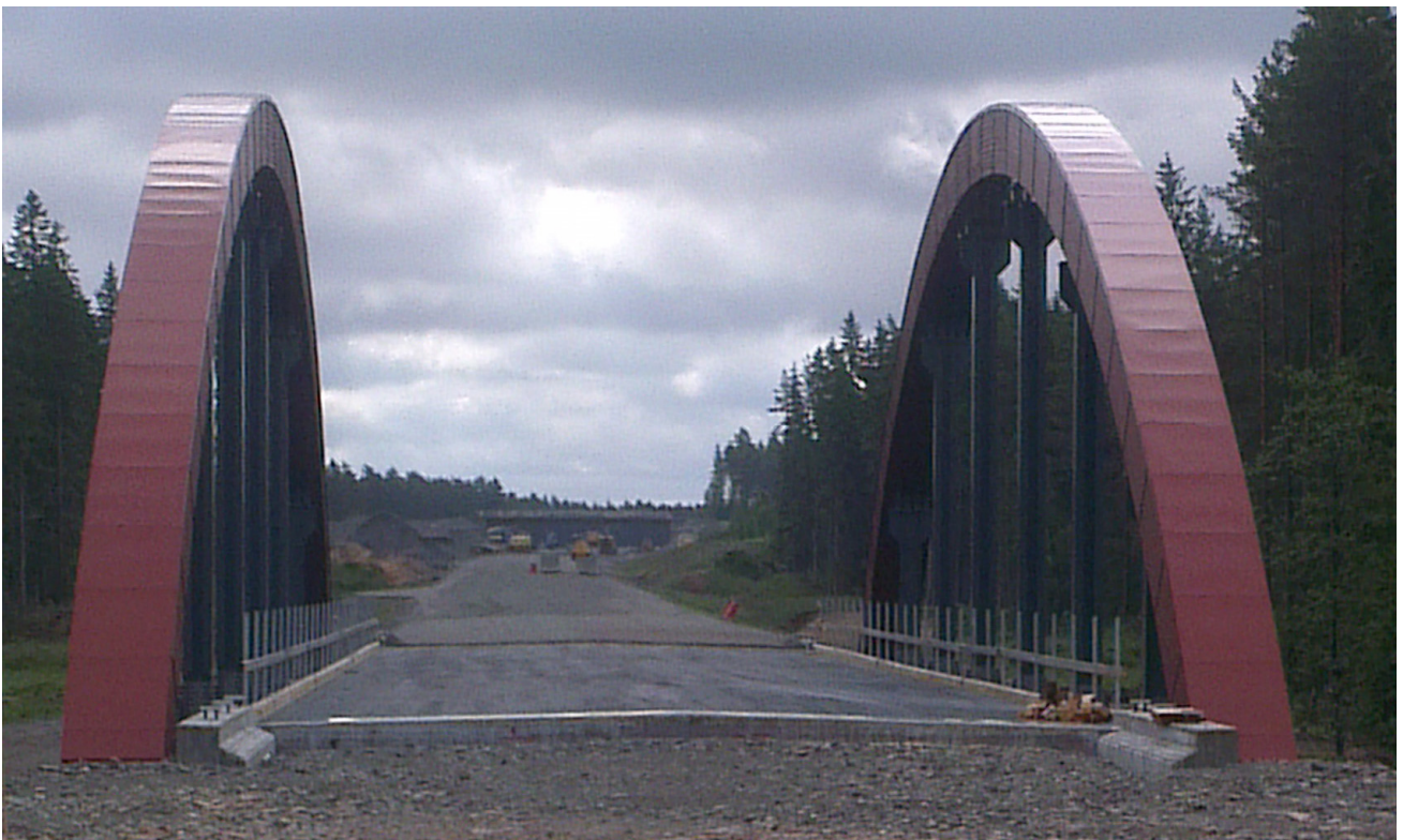
Fig. 15 View of the completed bridge without the asphalt surfacing.
