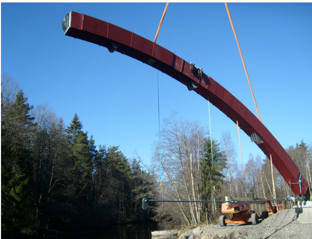
Fig. 11 First half of the arch lifted into position using a crane.
