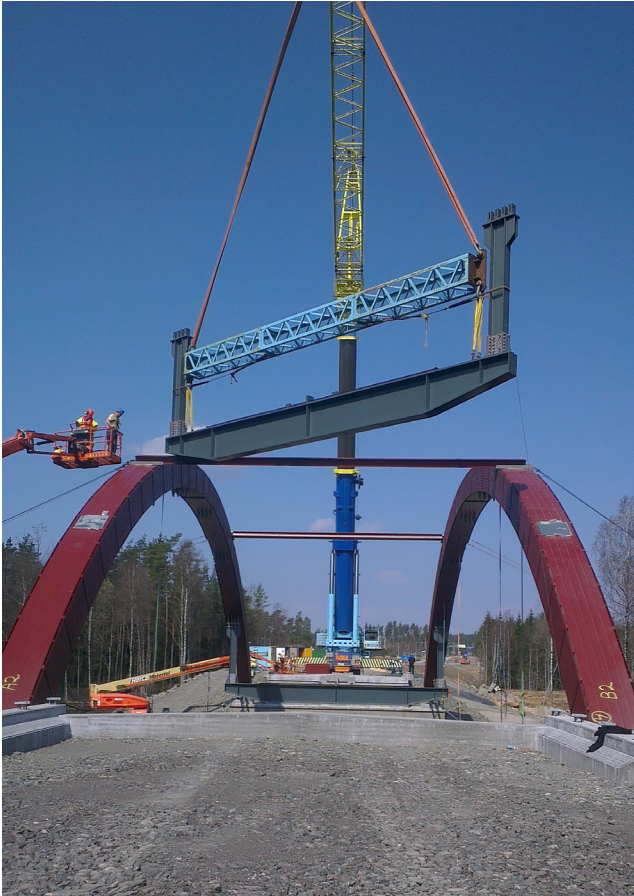
Fig. 13 The second frame is lifted into position.
