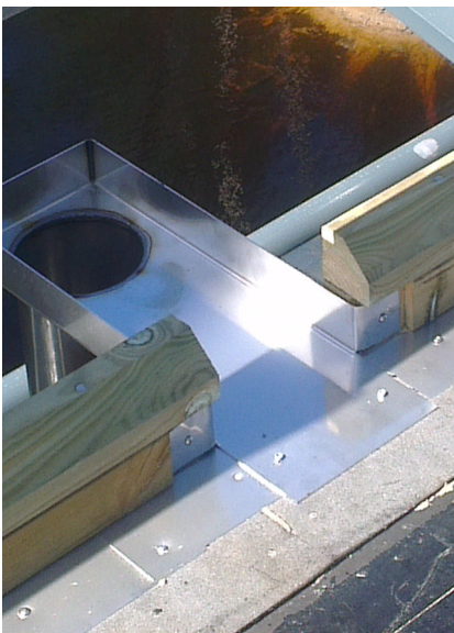
Fig. 7 Stainless steel inlet (before sealing board and asphalt are added)
