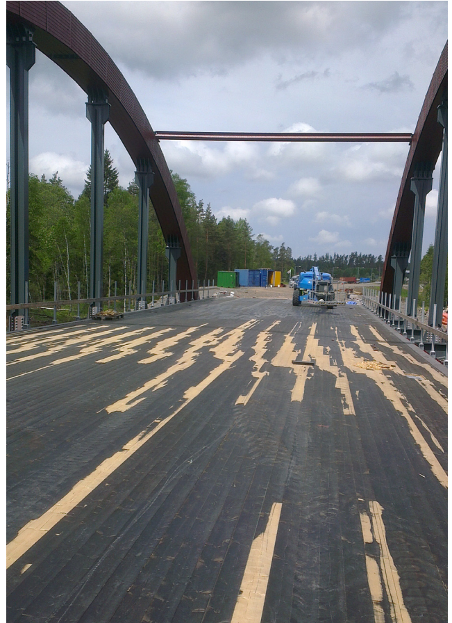
Fig. 14 SLT deck in position.
