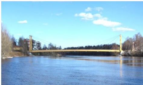
Fig. 1 Cable-stayed Timber Bridge of Skellefteå River
