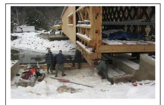
Figure 4 - Bridge being moved sideways into position atop the permanent abutments (with a bit of good-natured help from the owner of the construction company).
