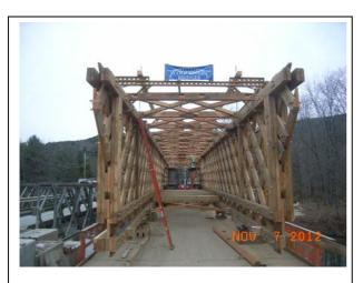
Figure 3 - Replacement timber bridge being built on a work platform bridge. The temporary vehicular bridge is at left in this photo. They were racing to beat bad weather, but looking good.
