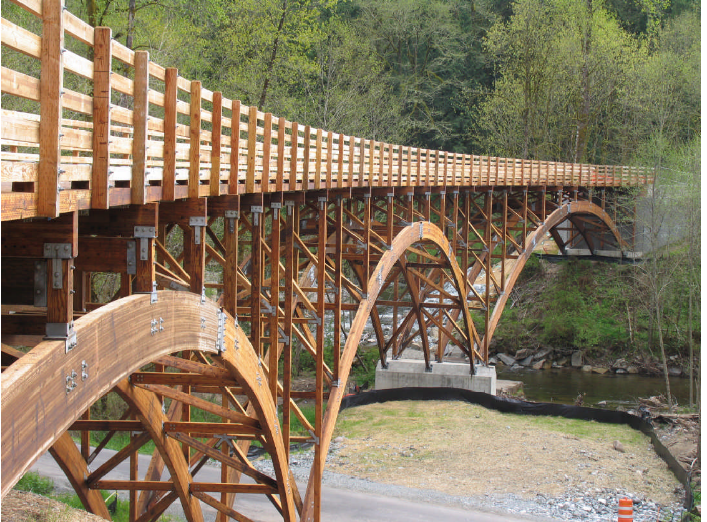
Figure 6. Lower Burnett Road Bridge
