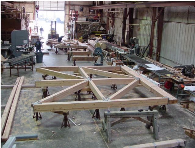
Figure 4. Preassembly of timber bents
