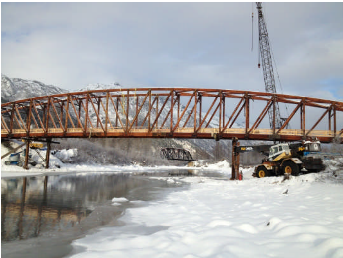
Figure 8. Completed bridge before removal of shoring
