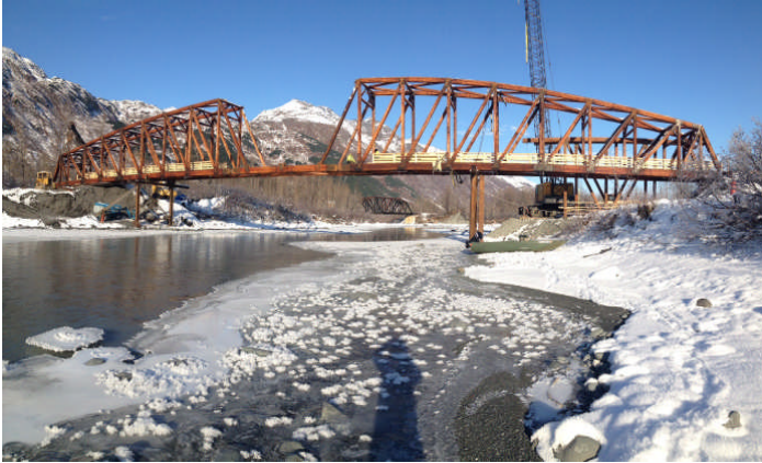
Figure 7. Piece-by-piece installation of the center truss section
