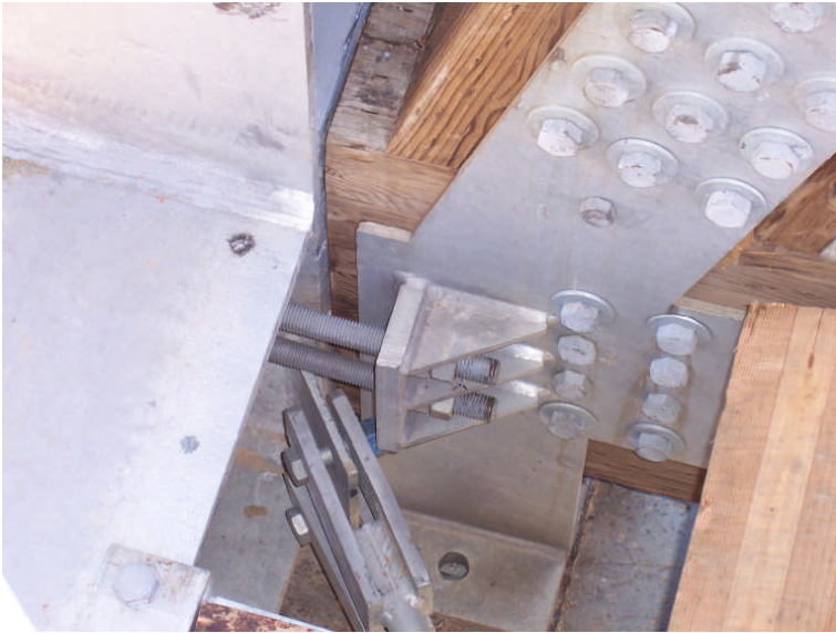
Figure 2. Tension/compression connection at pier
