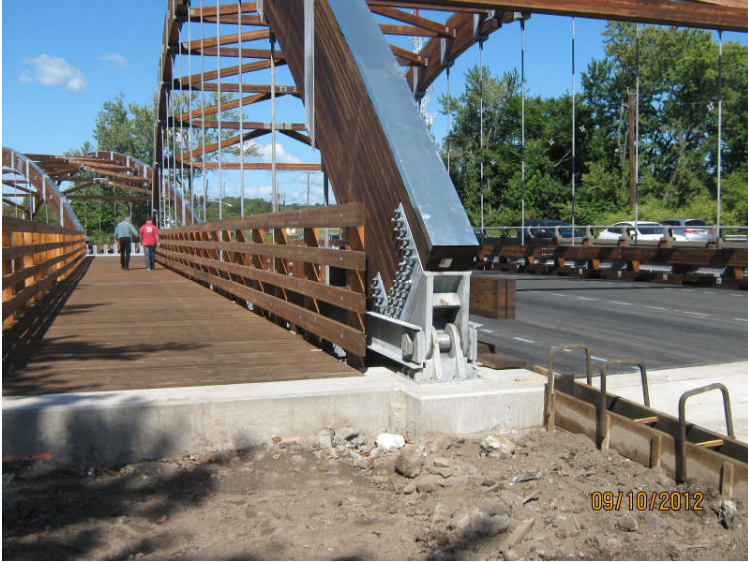
Figure 10. Tension tie channels connected to heel assembly
