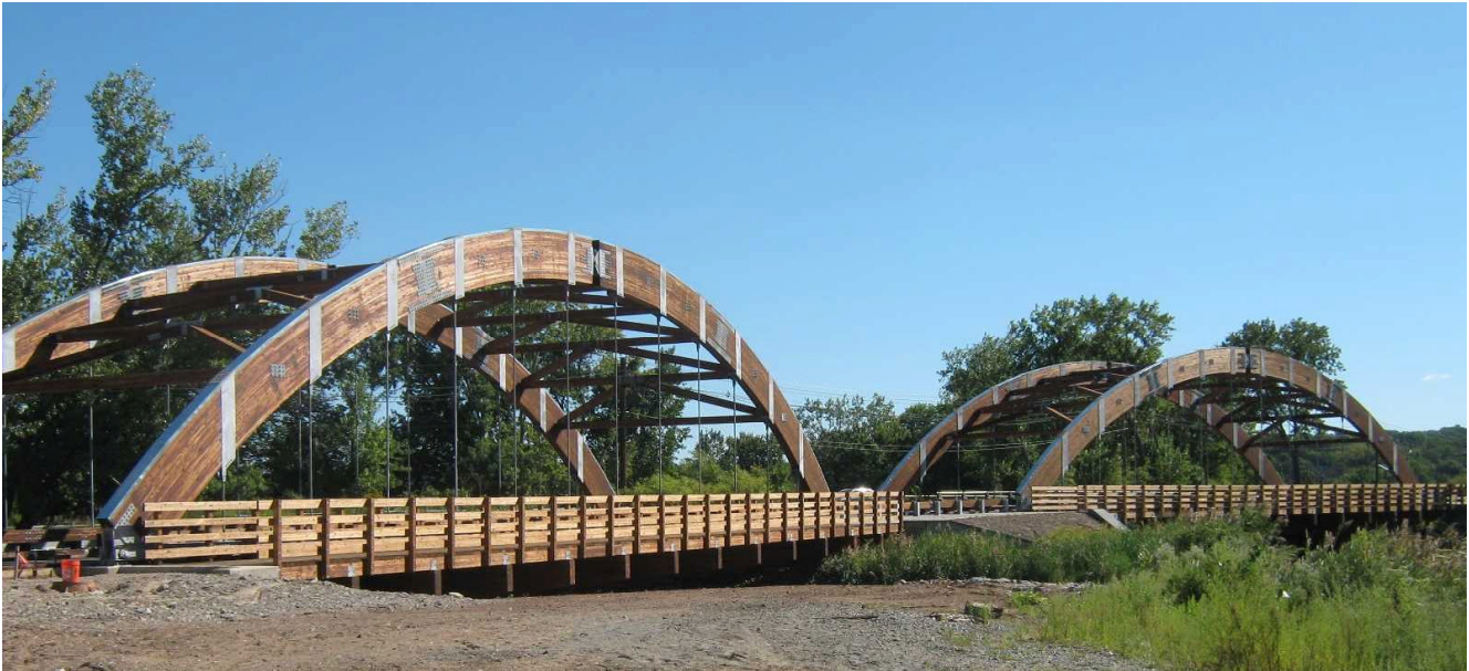
Figure 11. Completed Overpeck Park bridges
