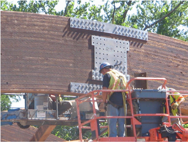
Figure 9. Workmen installing moment splice
