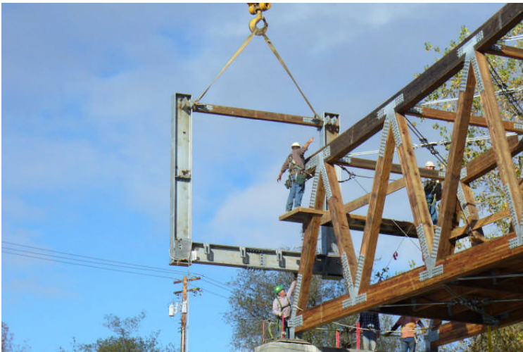
Figure 3. U-shaped, moment-resisting frame at piers
