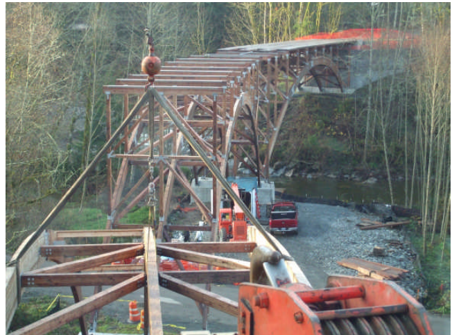
Figure 5. Installation of timber bents
